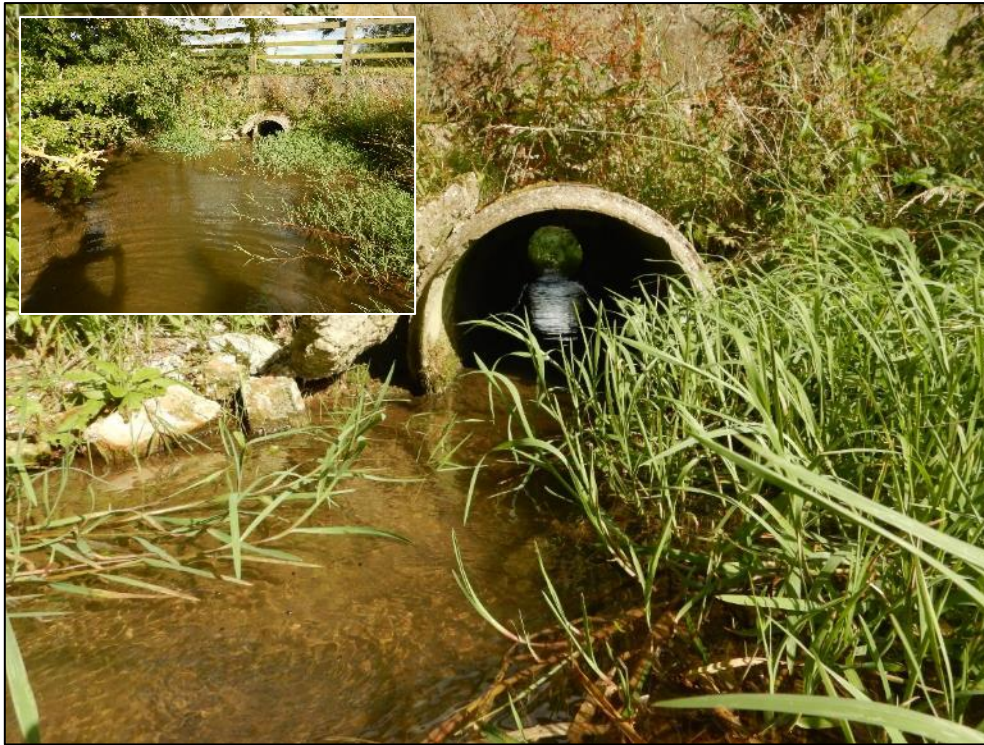
Pic 53 – Concrete culvert pipe (0.7m diameter) passable on day of visit but would become more challenging in high flows. The pool downstream is ~0.5m deep and is where trout (along with minnows in May 2024) had been seen in the past. This location is above the point of recent improvement work so the walkover ended (///sometimes.magma.clarifies). Good trout habitat in the pool (inset picture).
