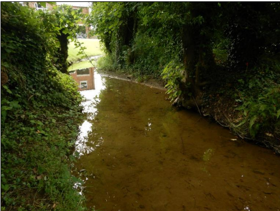
Pic 14 – A silted pool near private gardens was not fully accessed. If the pool was clear of silt, it would present fish holding habitat, no fish were observed. An appropriately located flow deflector could encourage cleansing of the pool (///lodge.forced.workroom). Adequate trout habitat where water depth above silt allows (but tidy gardens may limit fish-holding habitat).
