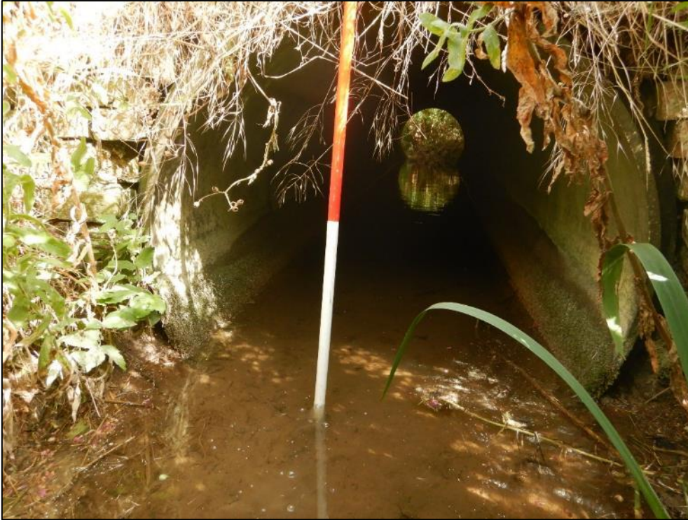
Pic 43 – Farm access culvert set below existing bed level presents no barrier to fish movements. Water vole feeding signs observed on flag iris (///loaded.strongman.turntable). Poor trout habitat.
