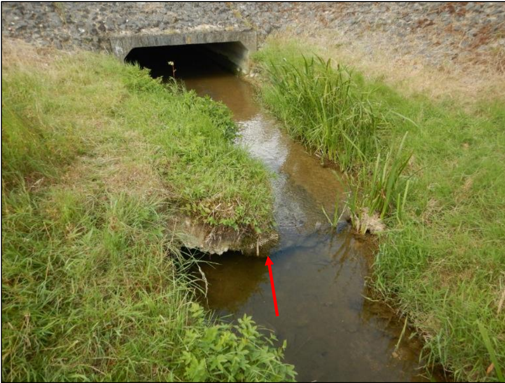
Pic 27 – An adult trout (>0.25m) took shelter beneath the dislodged concrete foundations (red arrow) of the Banovallum Gardens bridge (///freedom.laminated.public). Trout habitat is adequate.
