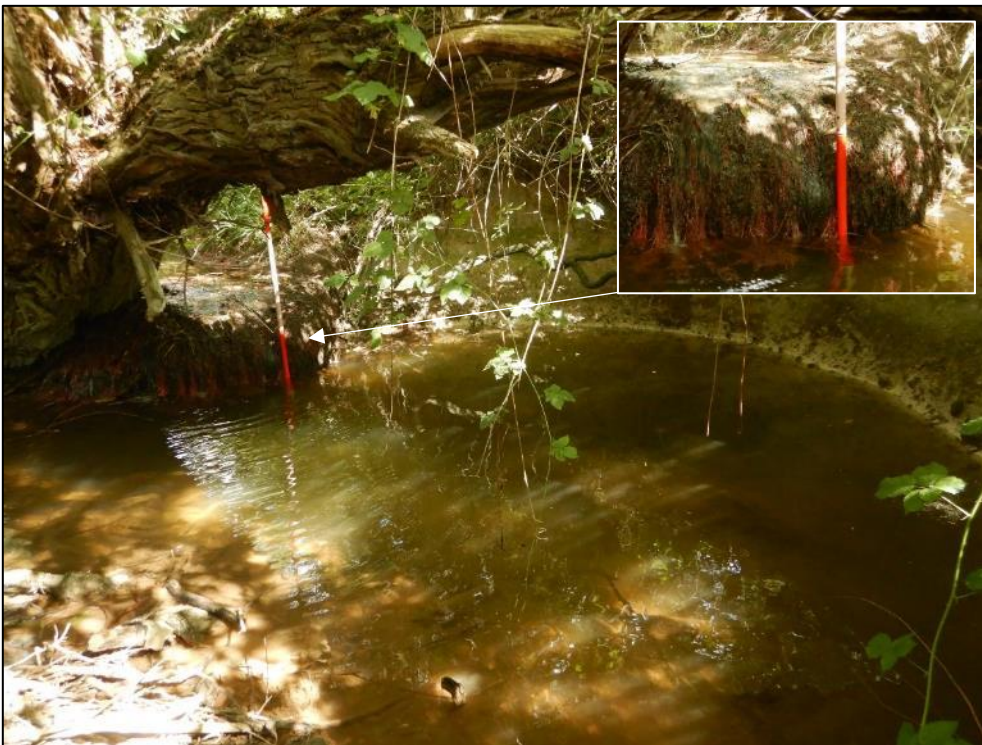
Pic 44 – Another plunge pool (~0.7m depth, ~3m width) from tufa forming over willow roots (indicating channel stability) focussing flow to the side of the pool and promoting scour. The restriction posed by the willow tree in combination with the drop presents further NFM, benefitting downstream communities and biodiversity. No fish were observed (///corded.reckoned.topic). Good trout habitat.
