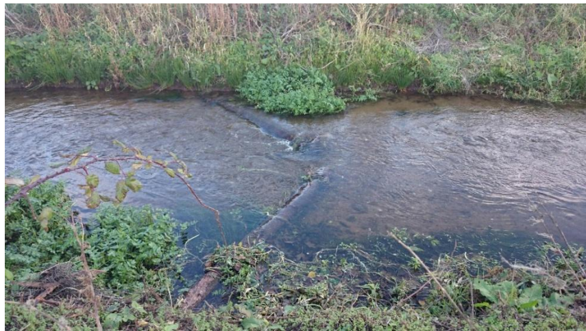
Figure 7 Upstream pointing pair of large woody deflectors recharging flow energy downstream.
