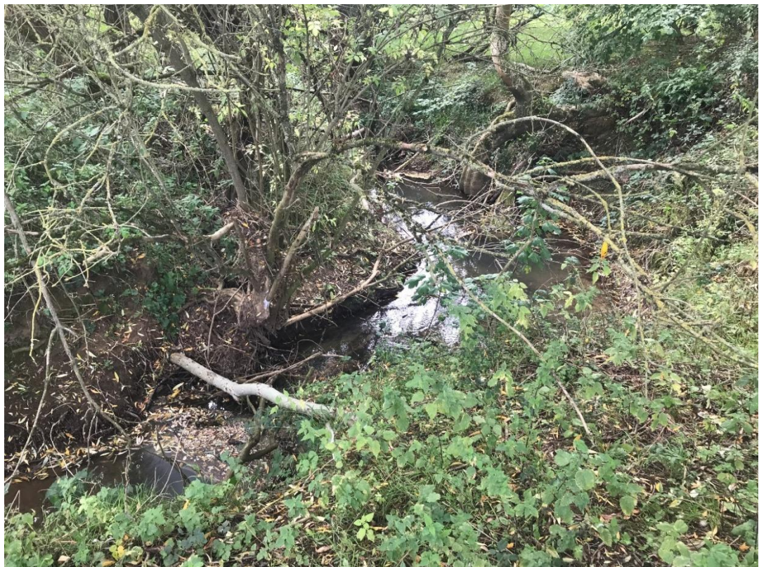
Photo 3 This continued into the first significant bend. One option for the whole of this reach upstream of the mill would be to utilise the material available in the adjacent wood to build some very large 'leaky dam' structures as a natural flood management measure. These would help slow the flow down during floods, back
