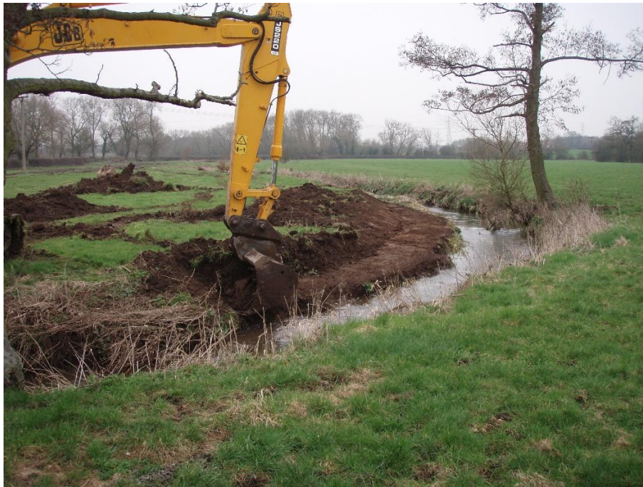
Figure 4 Bank reprofiling in action.
