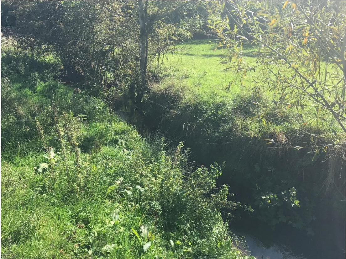
Photo 14 (52.026010 , -1.5422820) Highlighting the level of channel incision and the floodplain area as the valley floor opens out.
