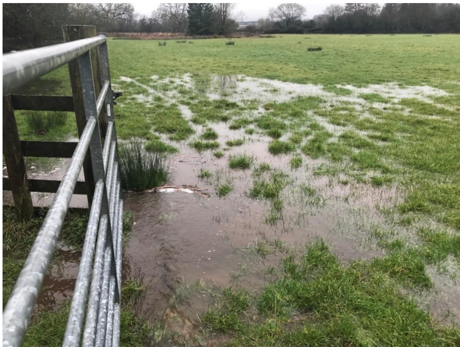
Photo 8 51.898494 , -1.7438661 A breach in the perched bank due to the river being elevated above the surrounding land. As this is just floodwater from the channel at high flow, it is not a huge issue for the river, simply creating wet meadow conditions of limited wildlife value. However, worth keeping an eye on as erosion could develop this into something more substantial over time.
