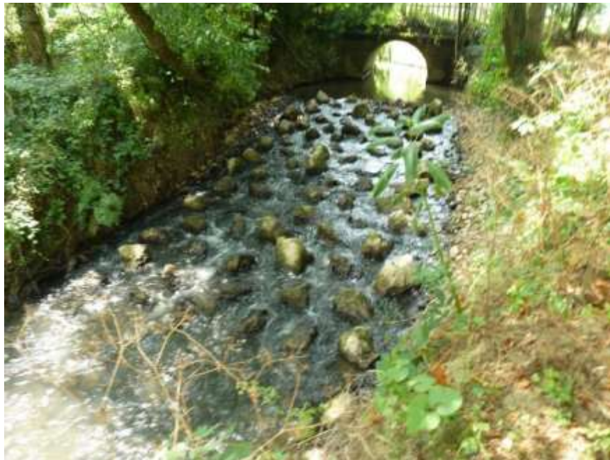
Figure 25: A rock ramp is an effective fish passage solution when a culvert cannot be modified with baffles or other easements, and a step up into it may need to be 'drowned out'. This example uses a series of erratic perturbation boulders to baffle the flow and ease fish passage.
