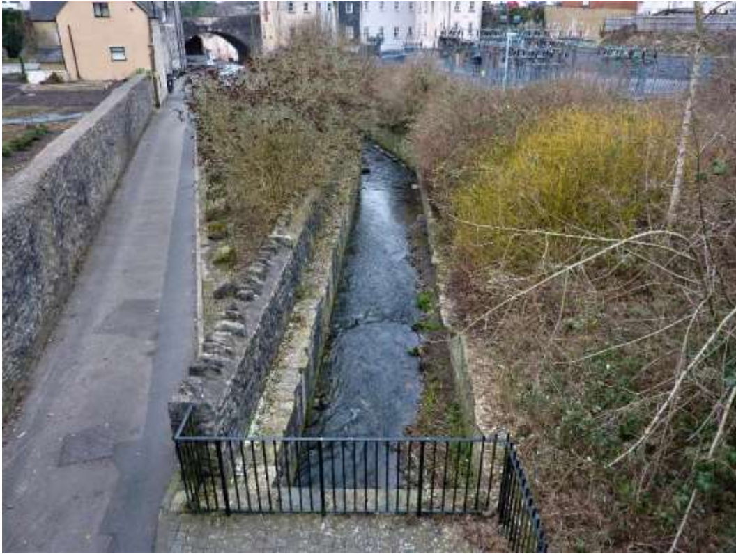
Figure 10: Looking downstream from the high footbridge over the River Sheppey and Lower Lane, with an unsightly transformer station on the RB, and the site of a potential pocket park on the LB
