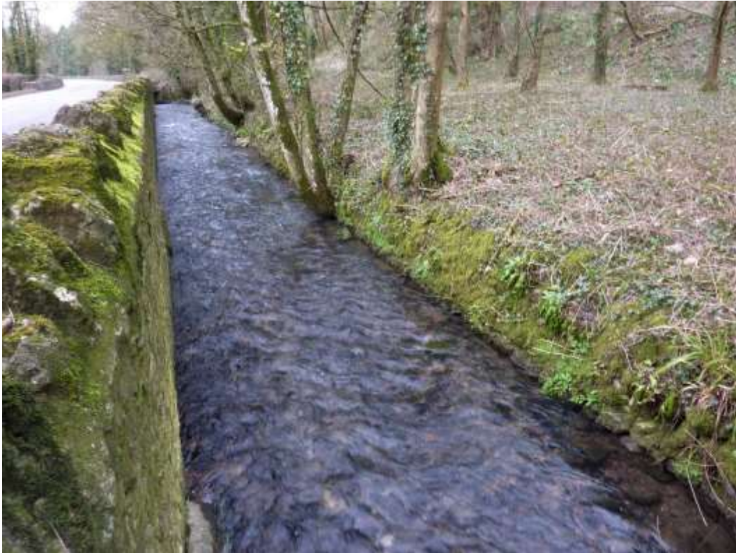
Figure 20: Approaching the Shepton Mallet STW, the river channel would benefit from added LWM for diversity and hydraulic roughness
