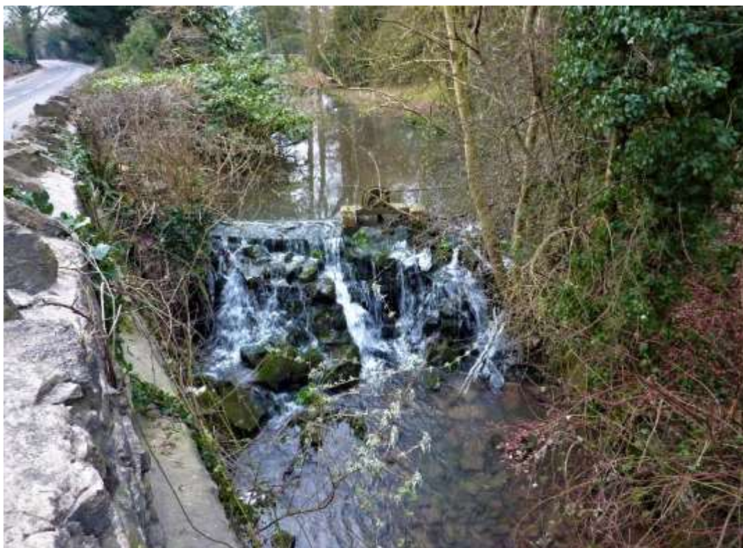
Figure 3: A redundant weir impounding c 120 m of the River Sheppey at Charlton
