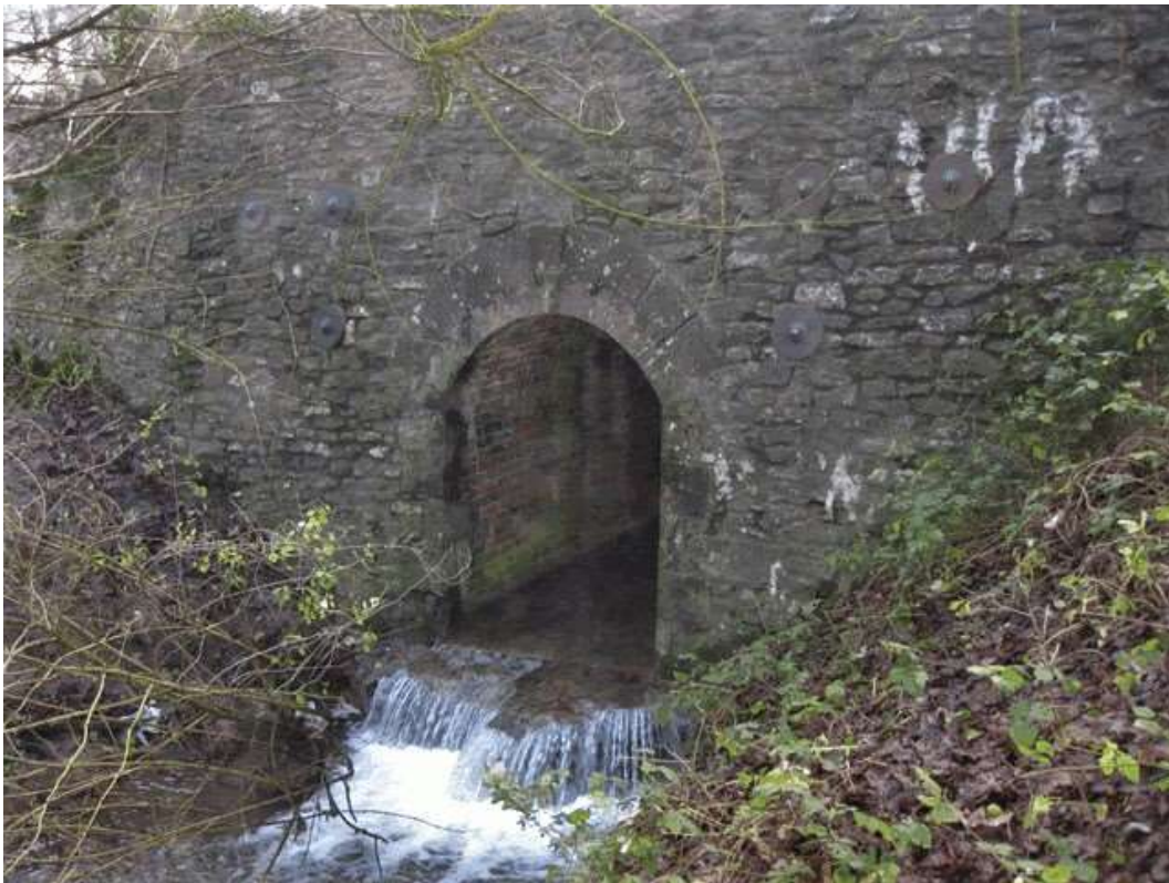
Figure 4: Shallow, impassable flow through the narrow bridge culvert under the A361 Charlton Road (Photo: Somerset Rivers: www.somersetivers.uk )
