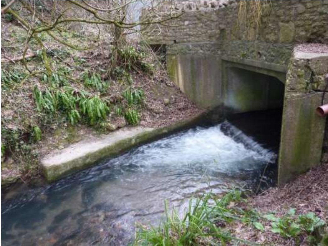
Figure 18: The culvert pool at the Darshill Mill access bridge
