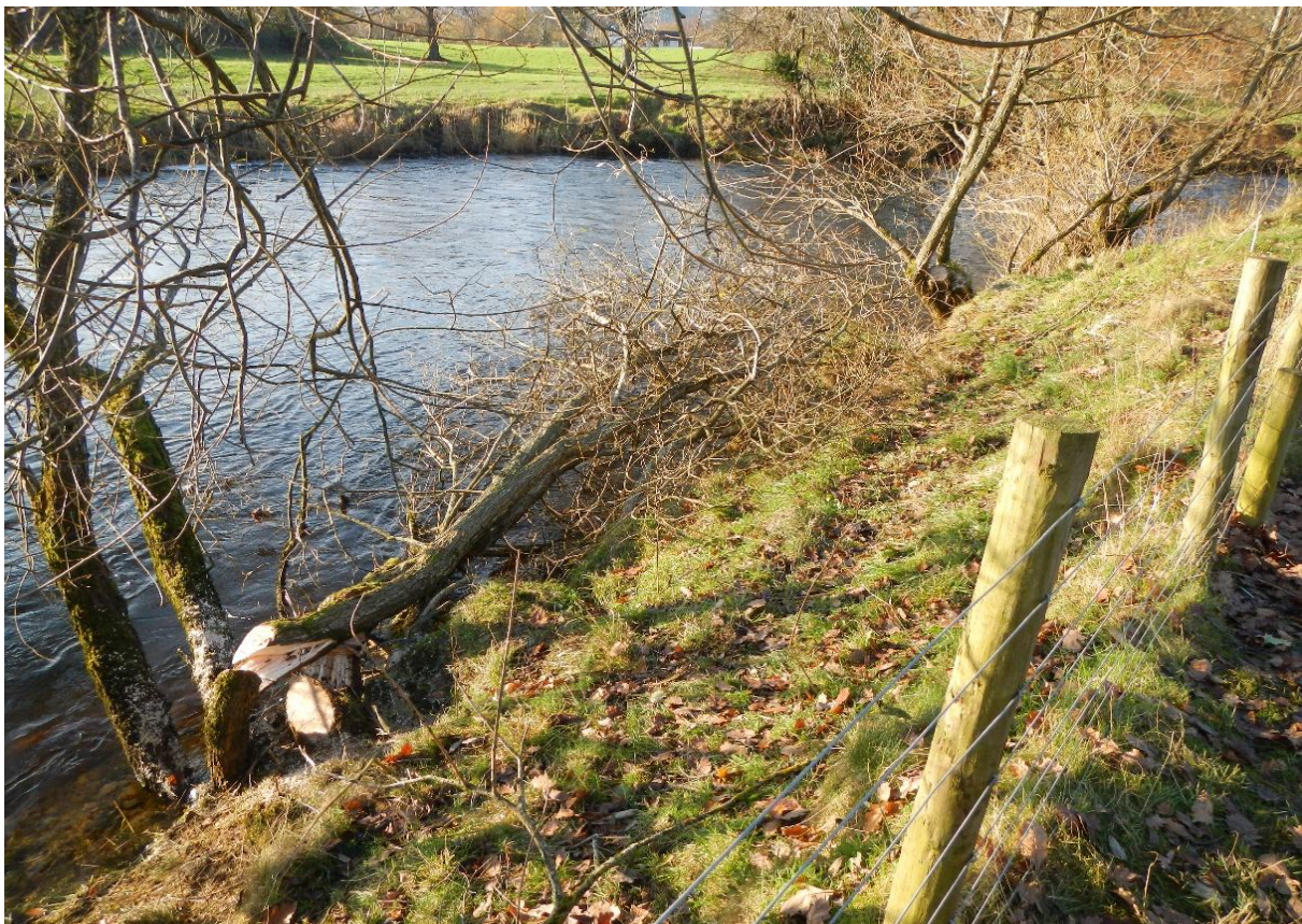
Fig 15. Two stems from a previously coppiced and hence multi-stem crack willow laid into the channel and aligned close to the bank to provide low / submerged cover. The living upright stems on the u/s side protect the hinge.
