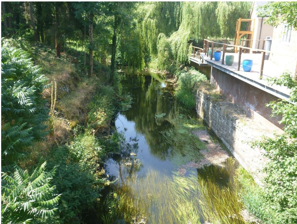
Photo 6 View d/s from Jubilee Bridge
