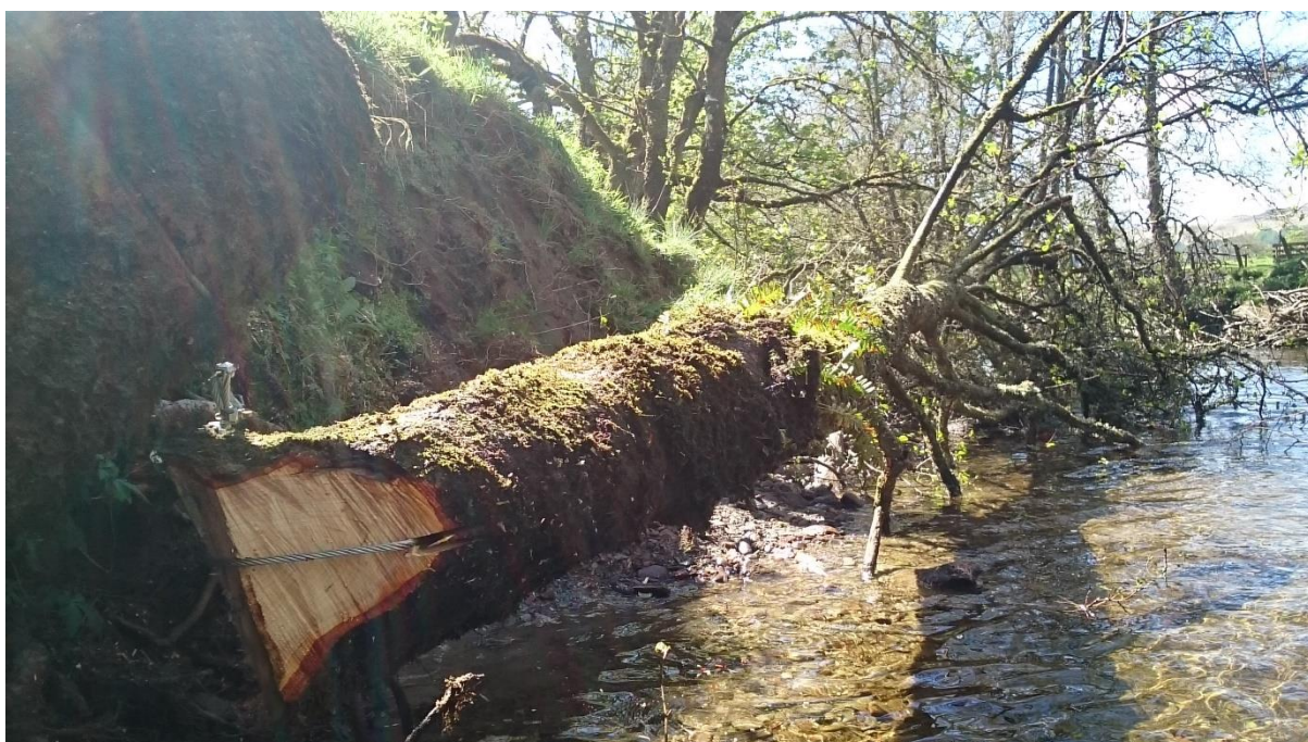
Figure 9: Cabled tree creating cover habitat as well as providing bank protection as a side-effect.
