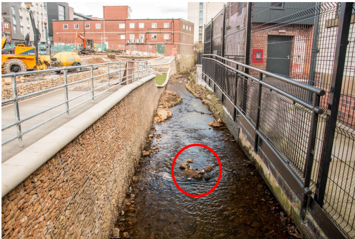
Figure 11: The same cluster of boulders shown in Fig.10 (circled) have caused a cobble and gravel riffle to deposit around and among that cluster in a walled section of steep, fast-flowing spate river.
