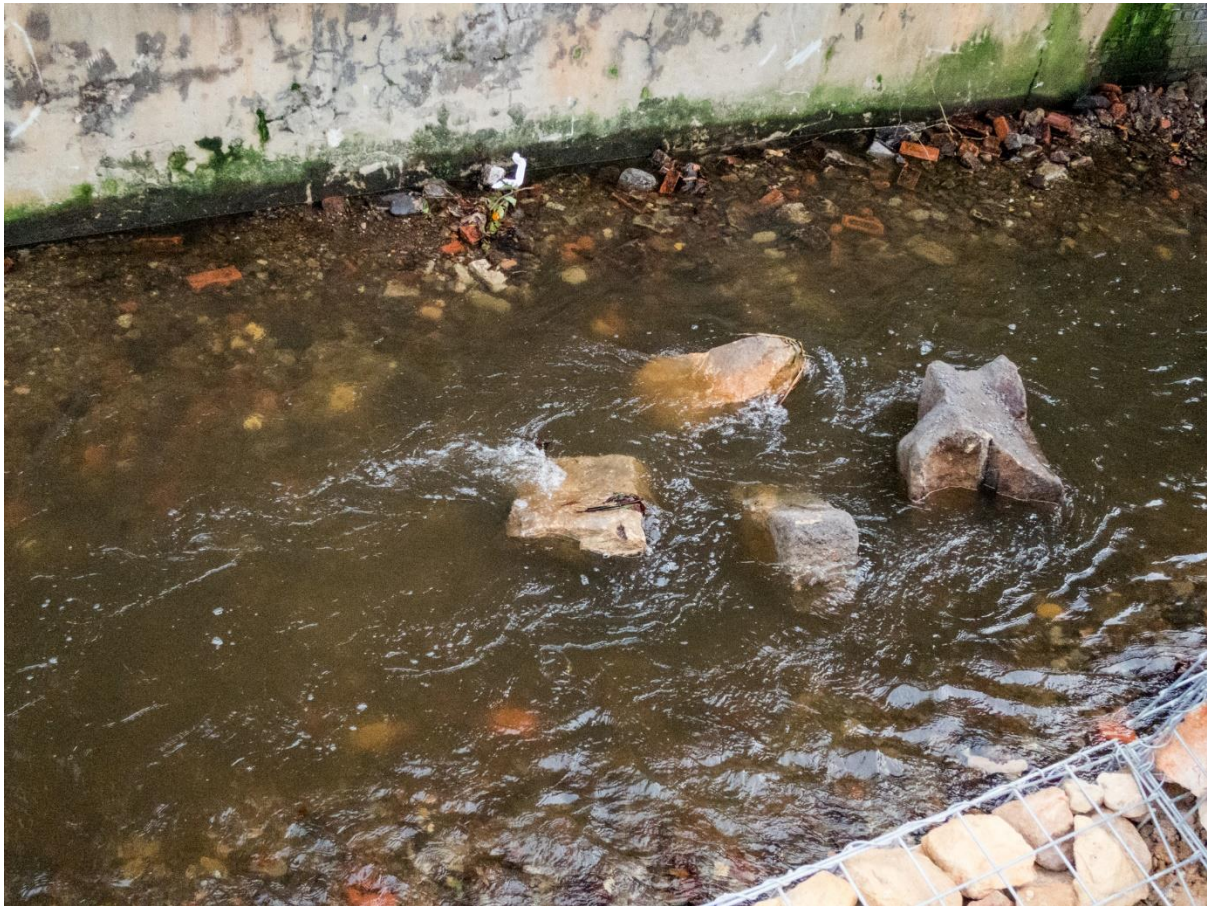
Figure 10: An example of one placement pattern of introduced boulders - where each rock represents a point making up a "diamond" shape. One of the corners of the diamond is pointing into the flow. The stream is flowing from the top right to bottom left corner of this picture.
