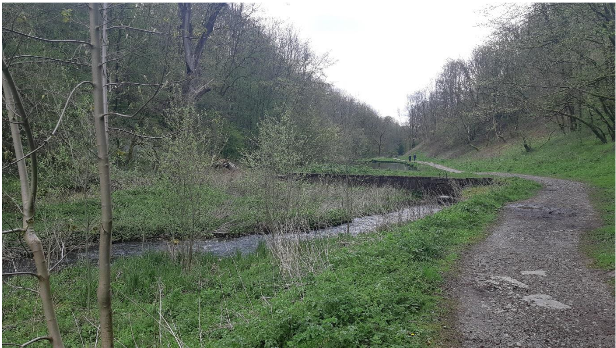
Figure 17: The dam wall for dam #2 – showing the former level of impoundment when the sluice was closed.
