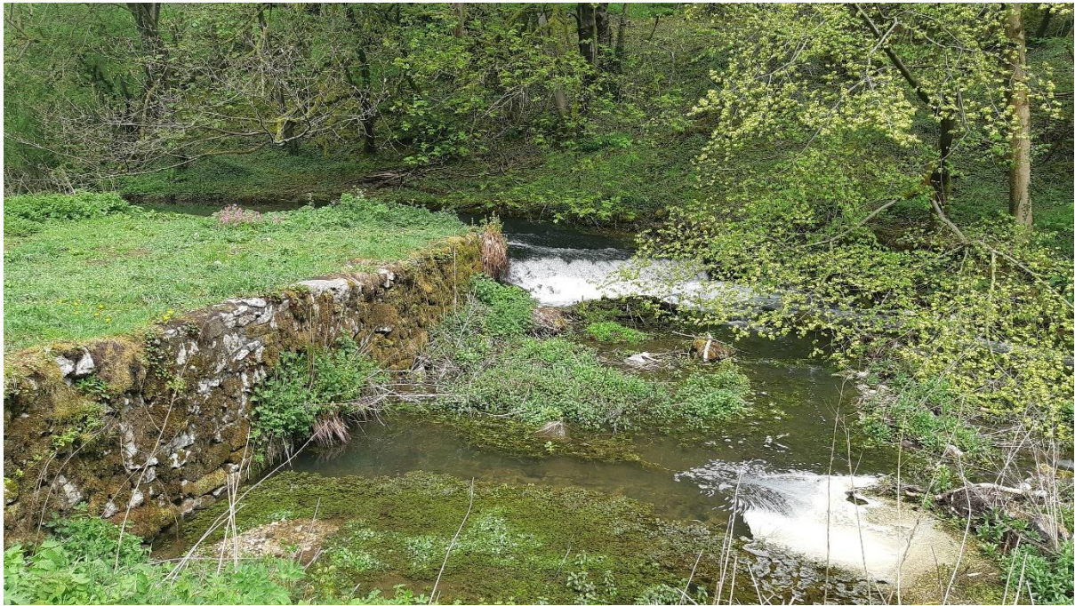
Figure 14: Overspill at the downstream end of dam #3.
