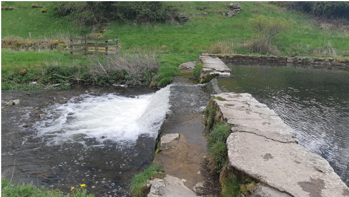
Figure 28: The weir that forms the swimming pool.
