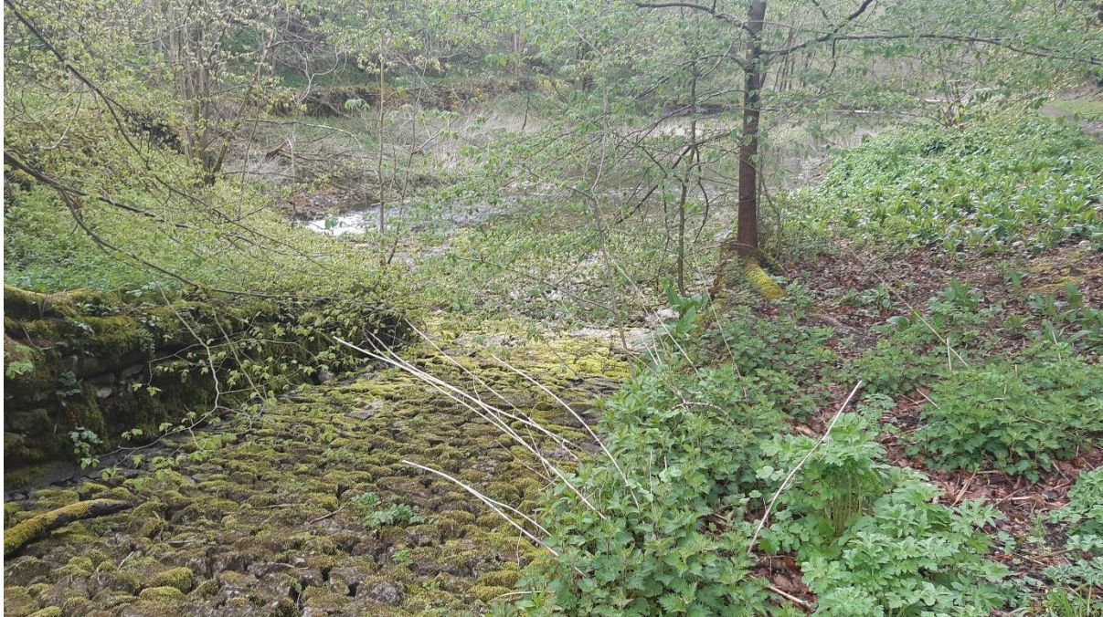
Figure 4: Cobbled overflow channel at the downstream end of the dam #5. Currently dry since the sluice gate bypasses this structure.
