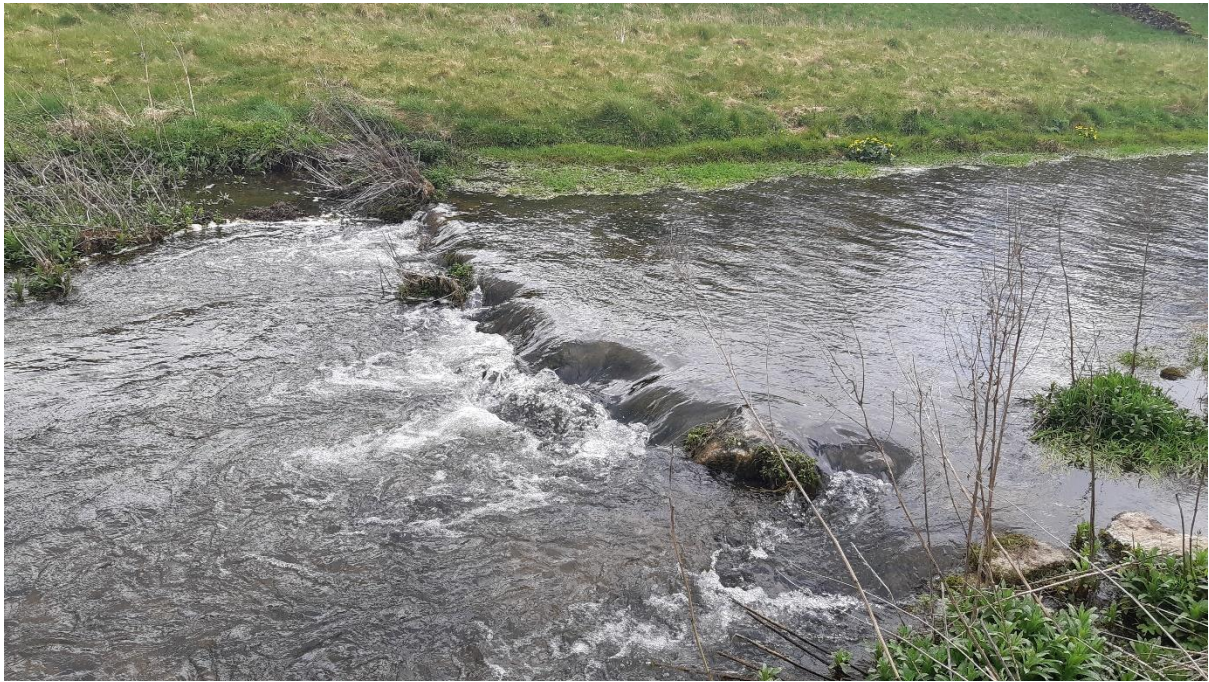
Figure 30: Boulder weir - amenable to simple block removal.
