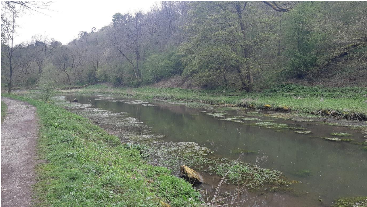
Figure 9: Central section of dam #4 facing upstream.
