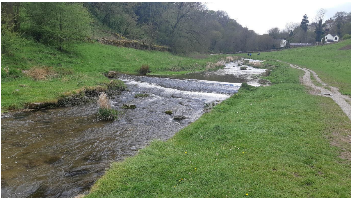
Figure 25: Apparent service pipe buried beneath a smooth, sloping weir-face.
