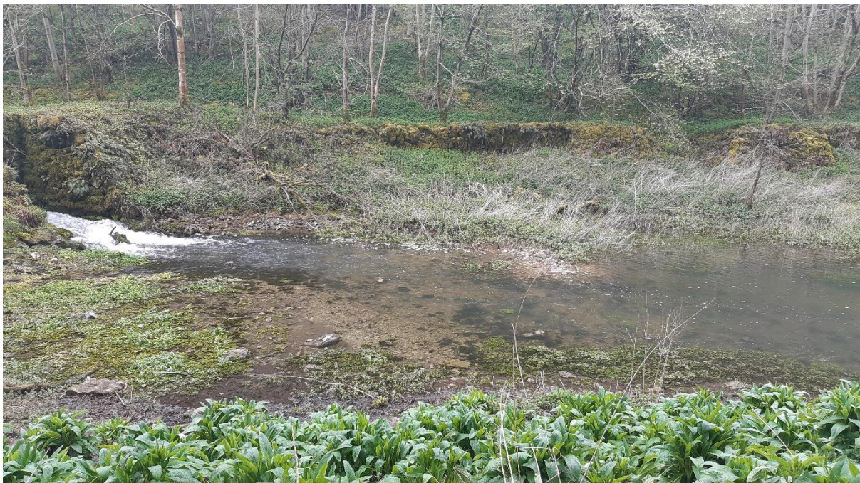
Figure 5: A shallow fan of gravel and cobble below the raised sluice draining dam #5.
