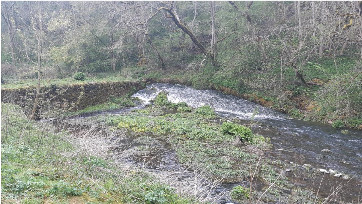
Figure 11: Overspill (in action) at the downstream end of dam #4 – there is potential for a baulk or other improvised baffle easement to be constructed on the sloping face.
