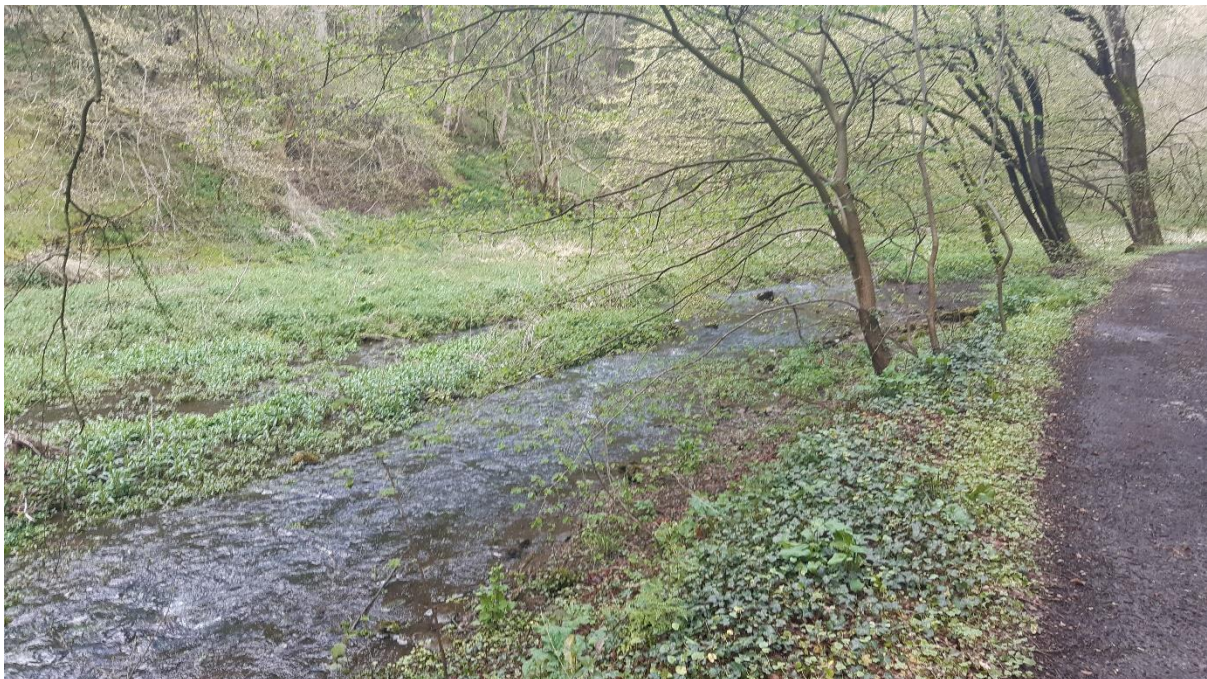
Figure 3: The dam furthest upstream on the Bradford - showing the condition with the sluice raised (and hence the “pond” is drained).
