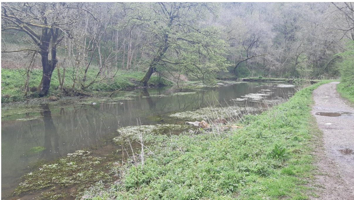
Figure 10: Dam #4 facing downstream.
