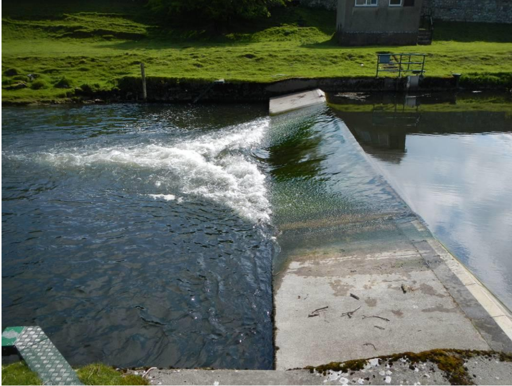
Figure 10. Bela Sit, flat-V gauging weir, posing a significant obstacle to fish movement in most flows.
