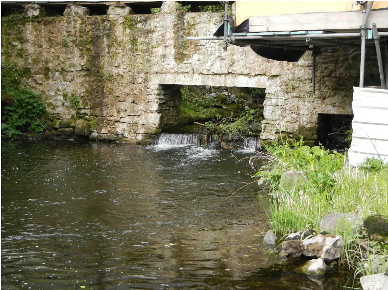
Figure 27. Poor attraction flow to the fish pass, exacerbated by debris blockage in the pass.
