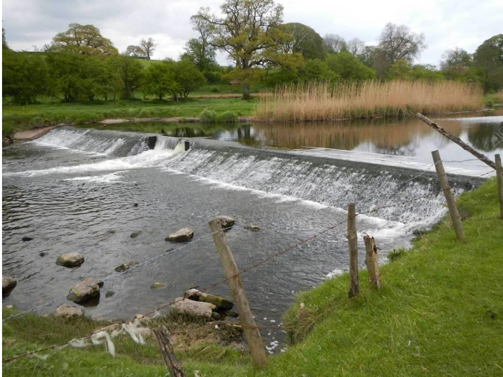
Figure 12. Tidal Weir, which will provide an obstacle to fish in low water, until it is drowned out by high spring tides, with a potential to significantly delay fish ascending the river.
