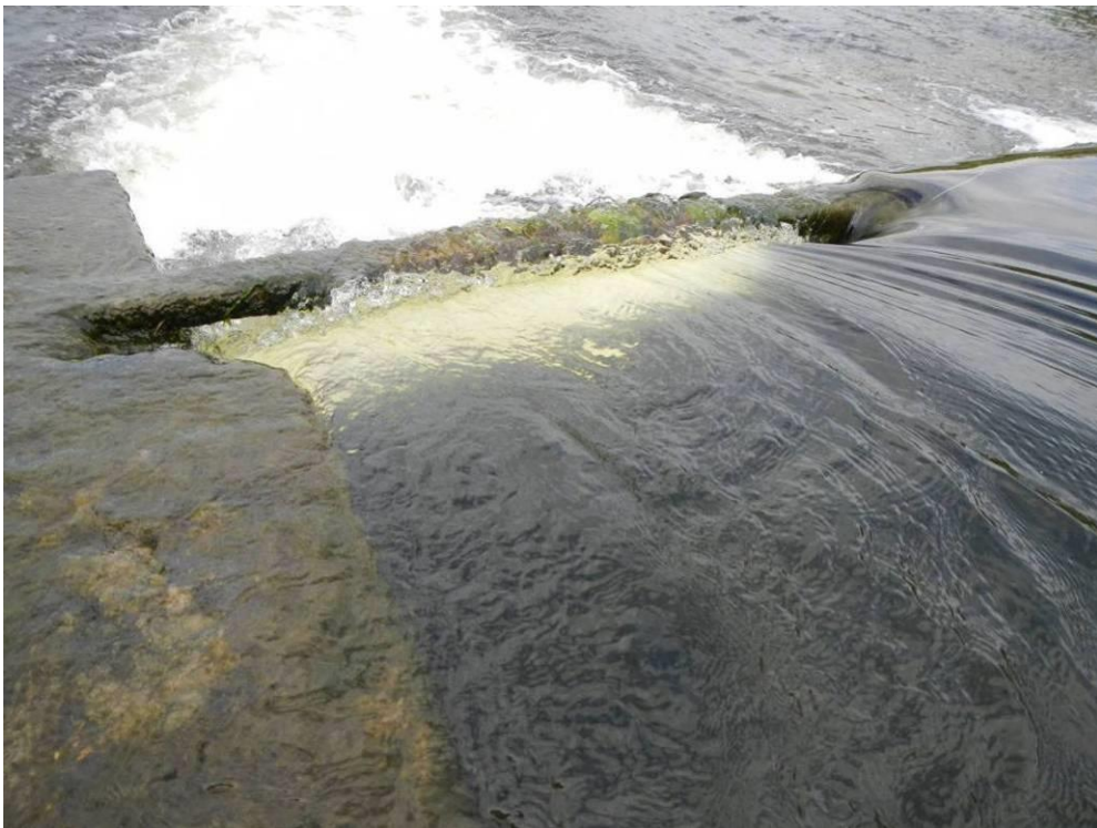
Figure 13. Slot through which fish passing the weir will have to travel in normal flows. The bar across the top of the gap further reduces the passability of the weir.
