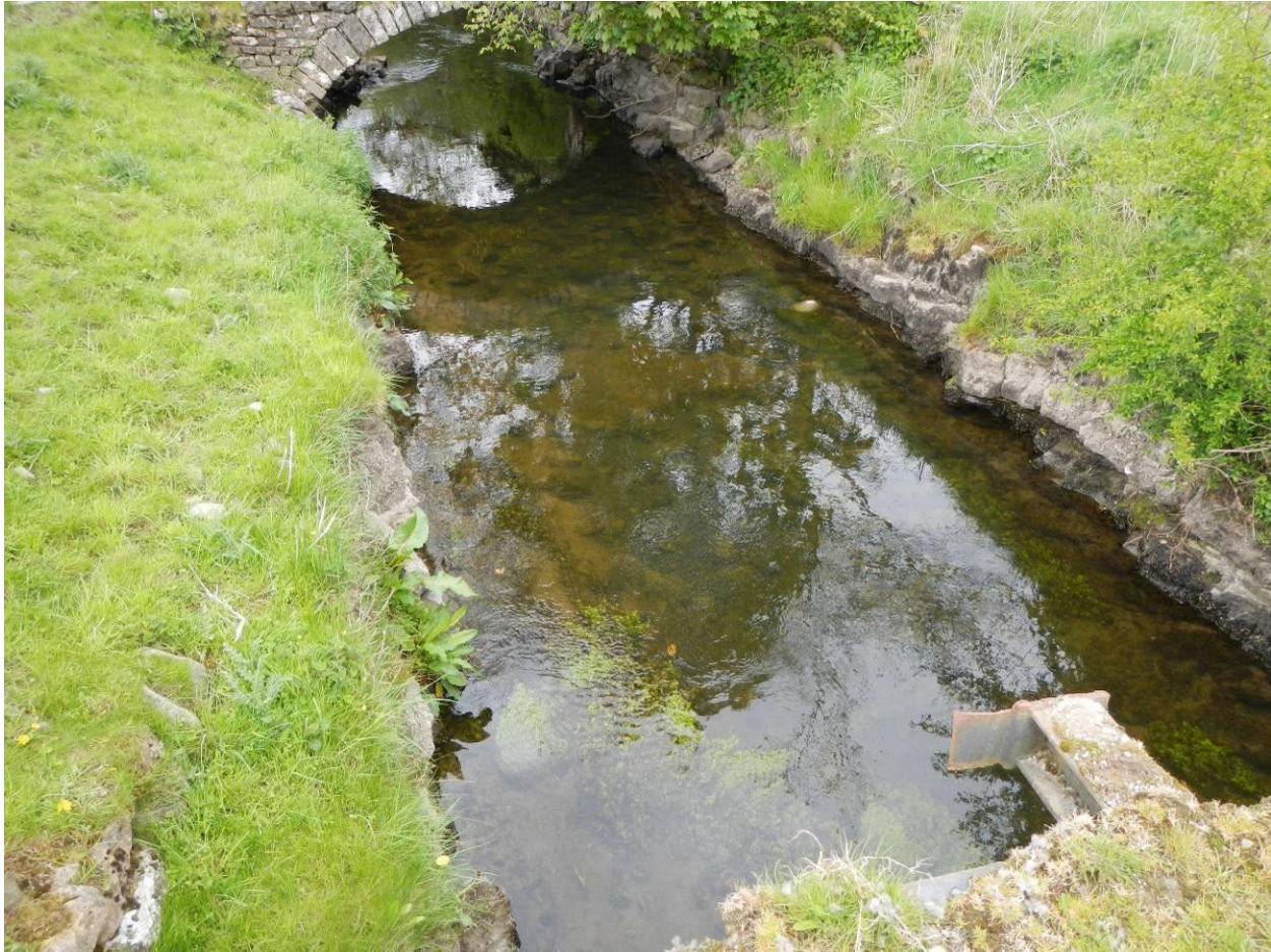
Figure 21. Section of the Holme Beck where the channel appears to have been carved out of the bedrock, leaving a featureless fixed cross section. Again, note sedimentation of the bed.
