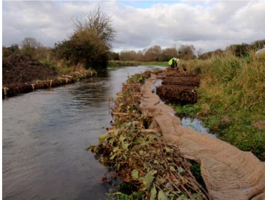
Figure 25. Bank creation using willow faggots and brush backfill. This example also includes the use of hessian or coir.
