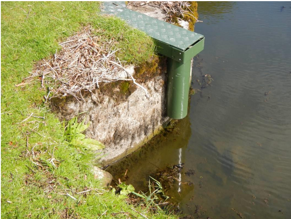
Figure 11. Upstream exit to eel pass, which is perched well above the water level and should be submerged.
