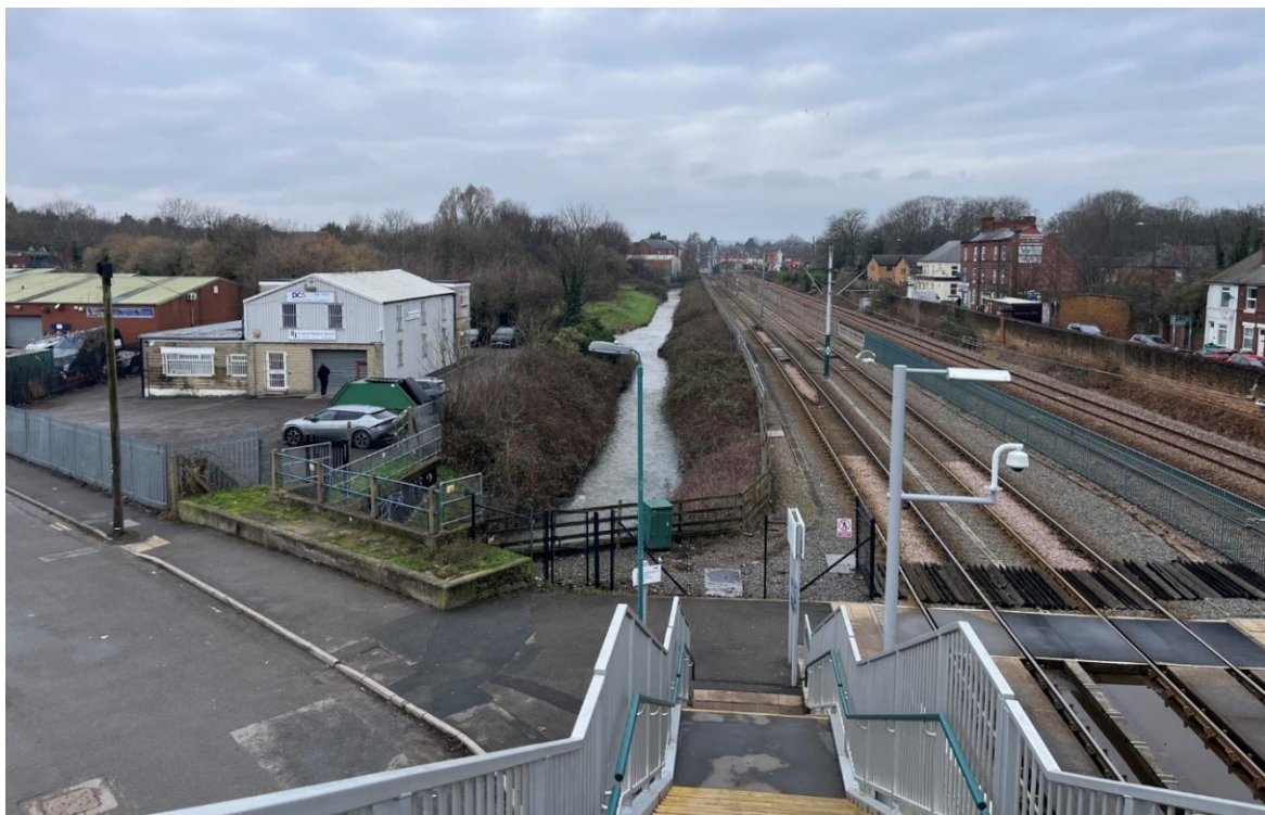
Figure 13: Illustration of straightened channel, constrained by tram/rail infrastructure along the LB at SK55237 43033. Note the slight widening of the channel, visible just above the street lighting fixture. Section part of Lincoln Street Open Space, looking upstream from Nottingham Road near Basford Tram Stop.
