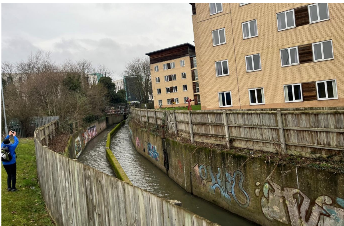
Figure 34: Central wall example at SK54933 40025 in a short, above-ground section of the Leen between Daisy Park student halls and railway line.
