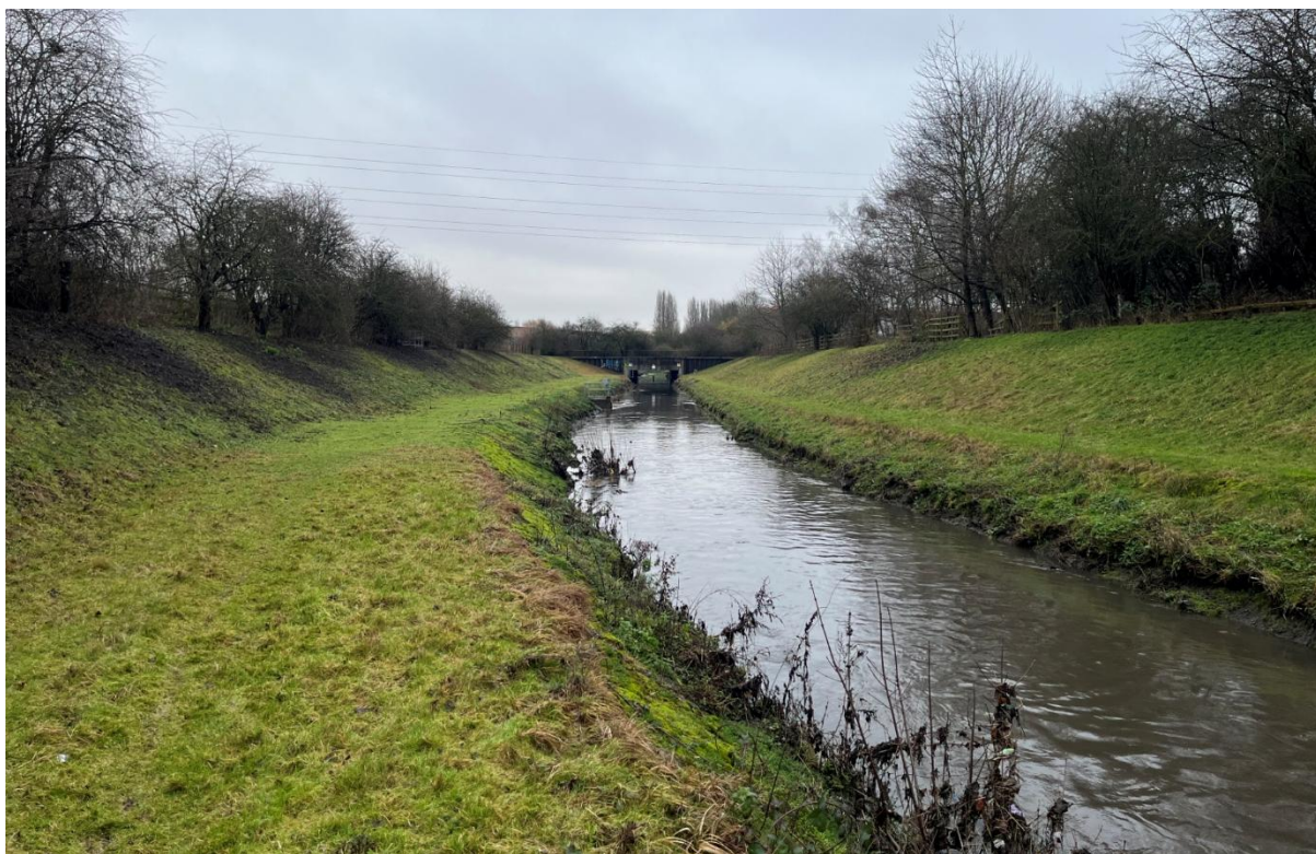
Figure 47: Facing downstream approximately 120m below Lenton Lane towards culvert. Note the significant additional floodwater capacity between the bridge upstream and culvert downstream. There is potential for re-meandering, more natural riverbed substrate introduction and in-channel large woody material here.
