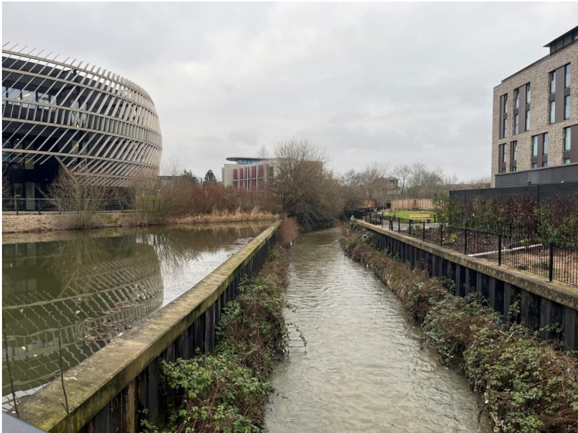
Figure 36: Elevated SuDS pond belonging to the Ingenuity Centre building (left), part of the University of Nottingham Innovation Park, adjacent to the River Leen at SK55085 39573.
