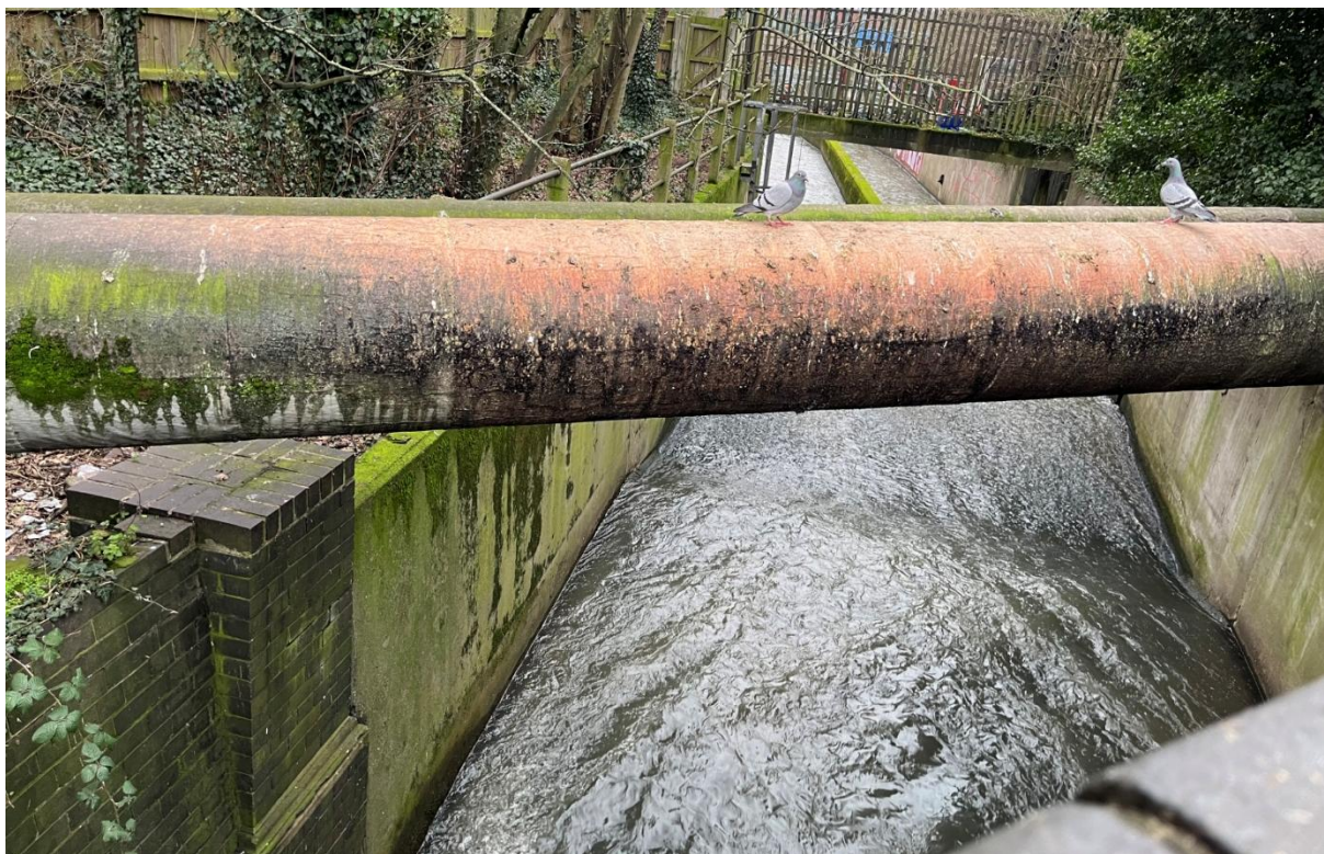
Figure 33: Weir at SK55038 40069 downstream of Wollaton Road with a smooth surface and laminar flow that creates a significant barrier to fish migration as well as substrate transport. Roughening the surface so as to promote accumulation of substrate would offer some improvement to habitat and connectivity.
