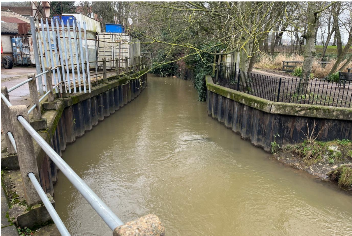
Figure 9: Sheet piling constraining channel at SK55114 43402 between factory and lake in a small park (Vernon Park) that currently suffers from antisocial drug use.
