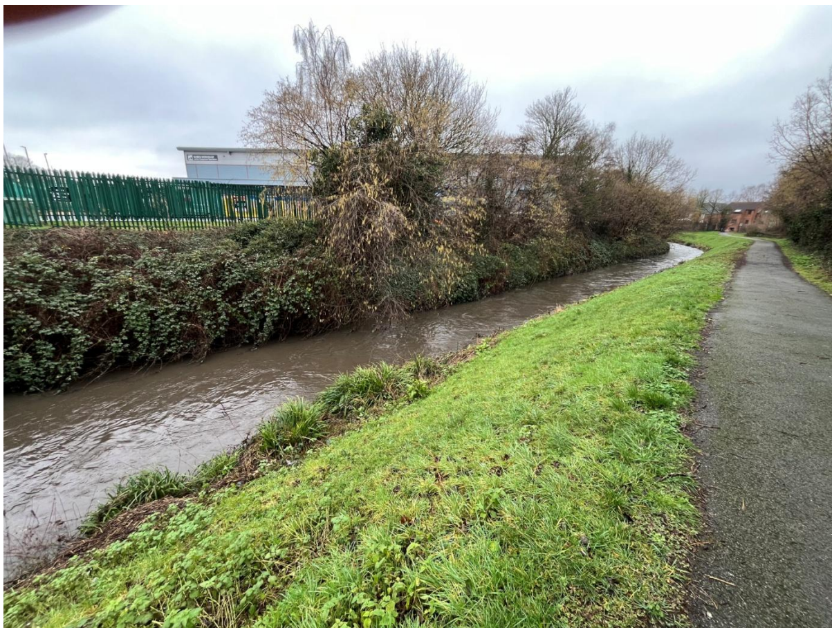
Figure 44: Left bank facing upstream just above the Willow Road bridge, Lenton area at SK55468 38520.
