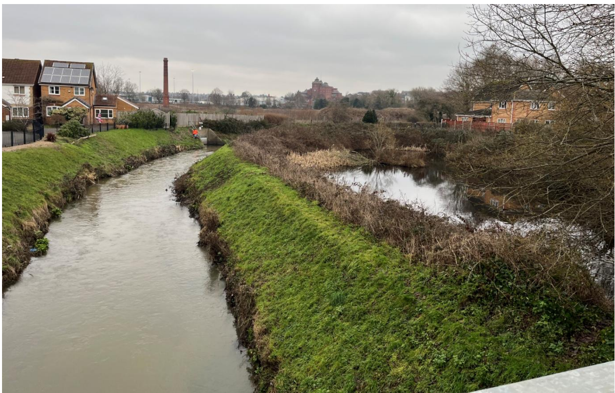
Figure 25: Facing upstream from Meadow Brown road (with steep-sided pond on LB; right of frame).
