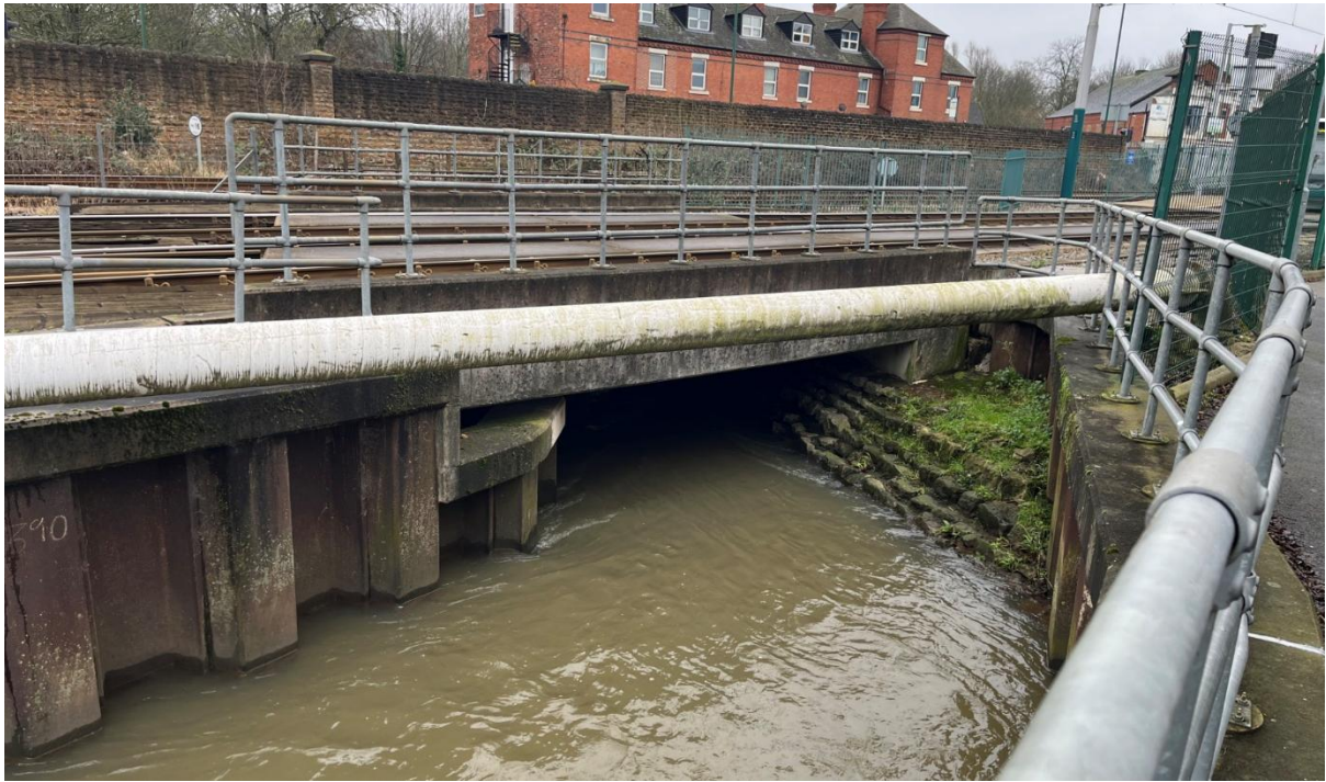
Figure 8: Hydraulic limit for the upstream reach imposed by the culvert beneath the rail infrastructure at SK54963 43420. Located near Vernon Road, upstream of Vernon Park.
