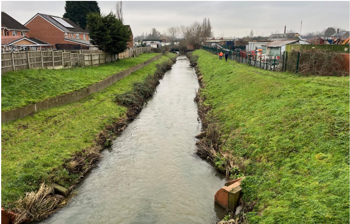
Figure 26: Facing downstream from Meadow Brown Road. Note the flood embankments and proximity to housing and business premises. In-channel large woody material, substrate-seeding and allowing riparian vegetation to grow would improve ecological potential here.
