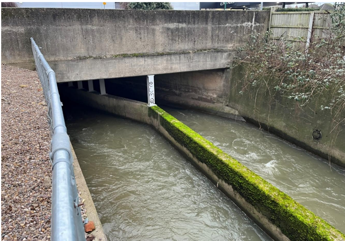
Figure 37: Culverted section emerging into completely straight concrete-walled channel with central concrete dividing wall at Triumph Road, SK55025 39327.
