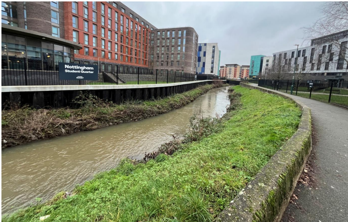
Figure 32: The degree of urban development lining the edges of the channel in these reaches presents huge challenges to river habitat improvement here. Sensitivities over flood risk do need to be balanced with a realistic assessment of the impact of allowing more structurally-diverse riparian vegetation to develop.
