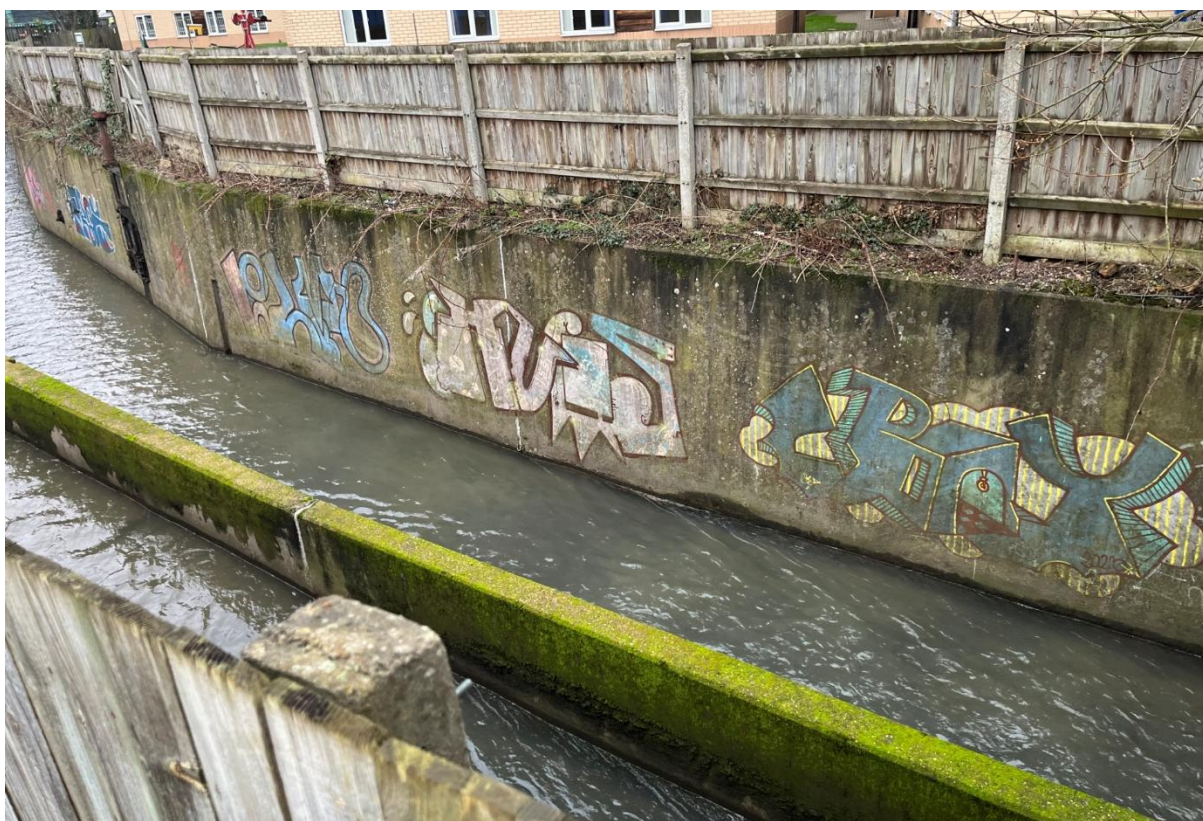
Figure 35: View of channel adjacent to Daisy Park student halls just as it passes over a small weir and into a culvert.
