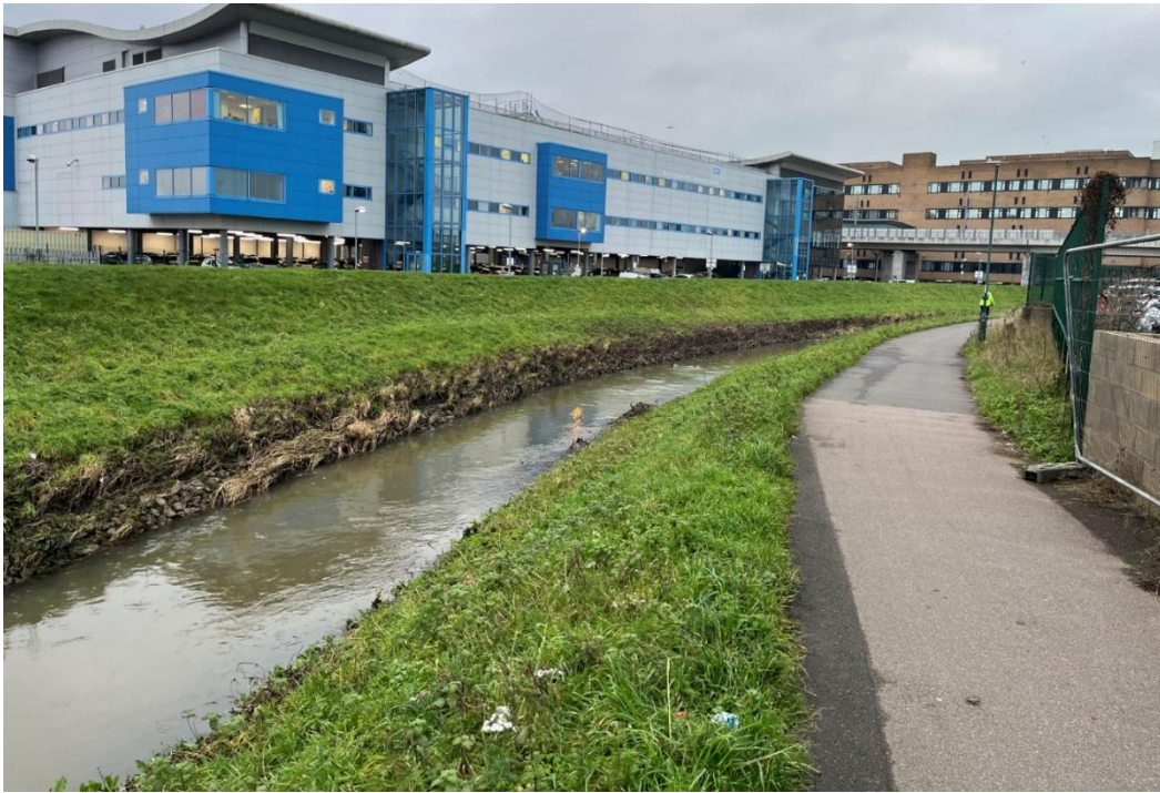
Figure 42: Just upstream of the next bridge downstream of Fig. 41 at SK55149 38644, opposite the Nottingham NHS Treatment Centre. Note a small amount of erosion on the opposite bank on the outside of the bend. The adjacent car park and degraded river corridor currently restricts the amenity value of the riverside to hospital patients and staff. Compare with Sheffield's pocket park creation at Matilda street for flood risk, public amenity and habitat improvement: https://www.wildtrout.org/wttblog/reducing-flooding-creating-urban-oasis-and-home-wild-trout
