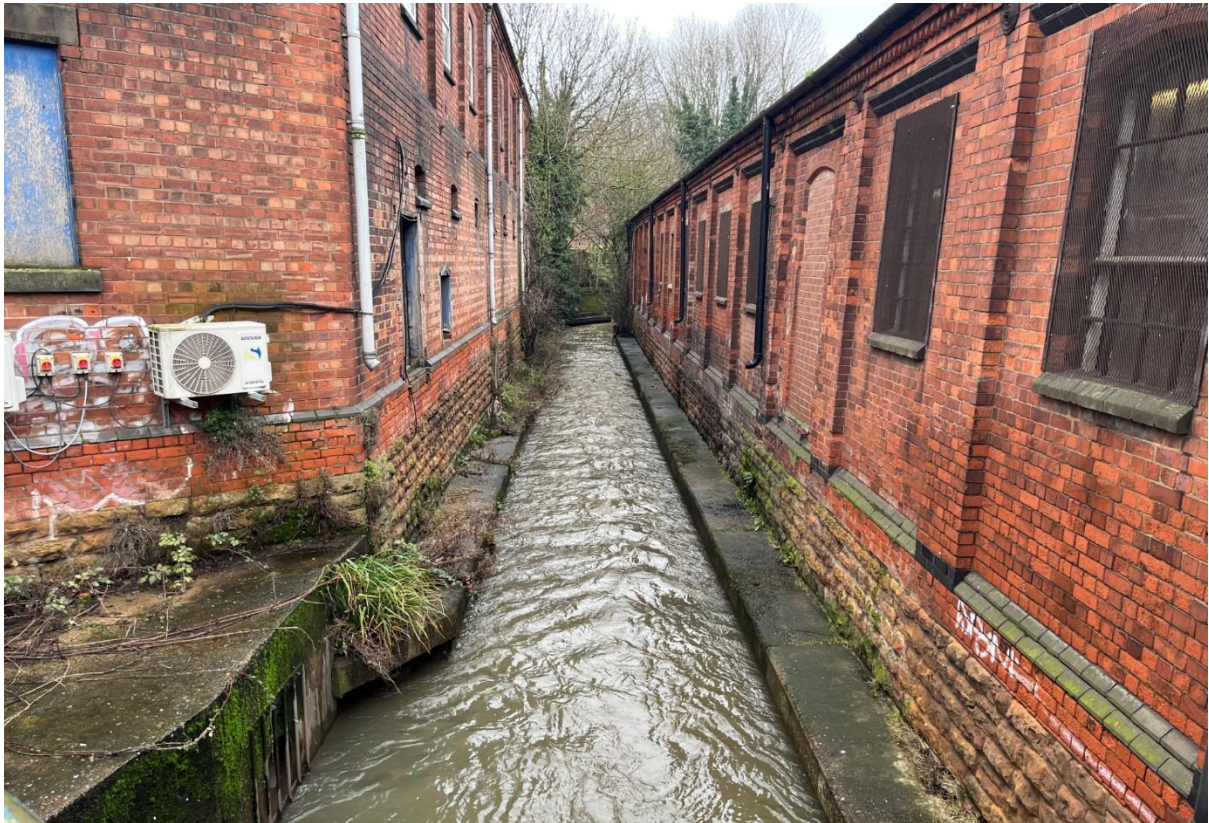
Figure 10: Constrained channel downstream of Southwark Street and feeding into the section shown in Fig. 9.
