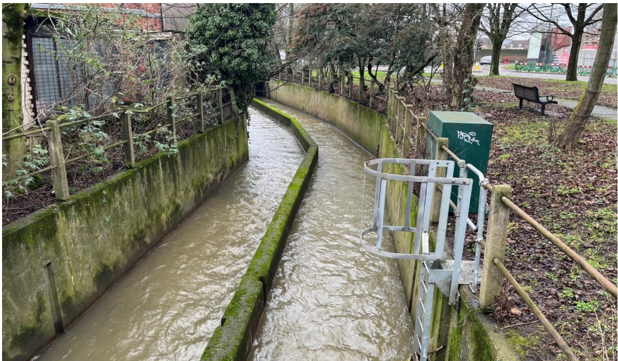
Figure 11: Typical example of central, channel-maintenance wall, plus access ladder, between factory and Vernon Park. Section between Vernon Road and Southwark Street, Basford.
