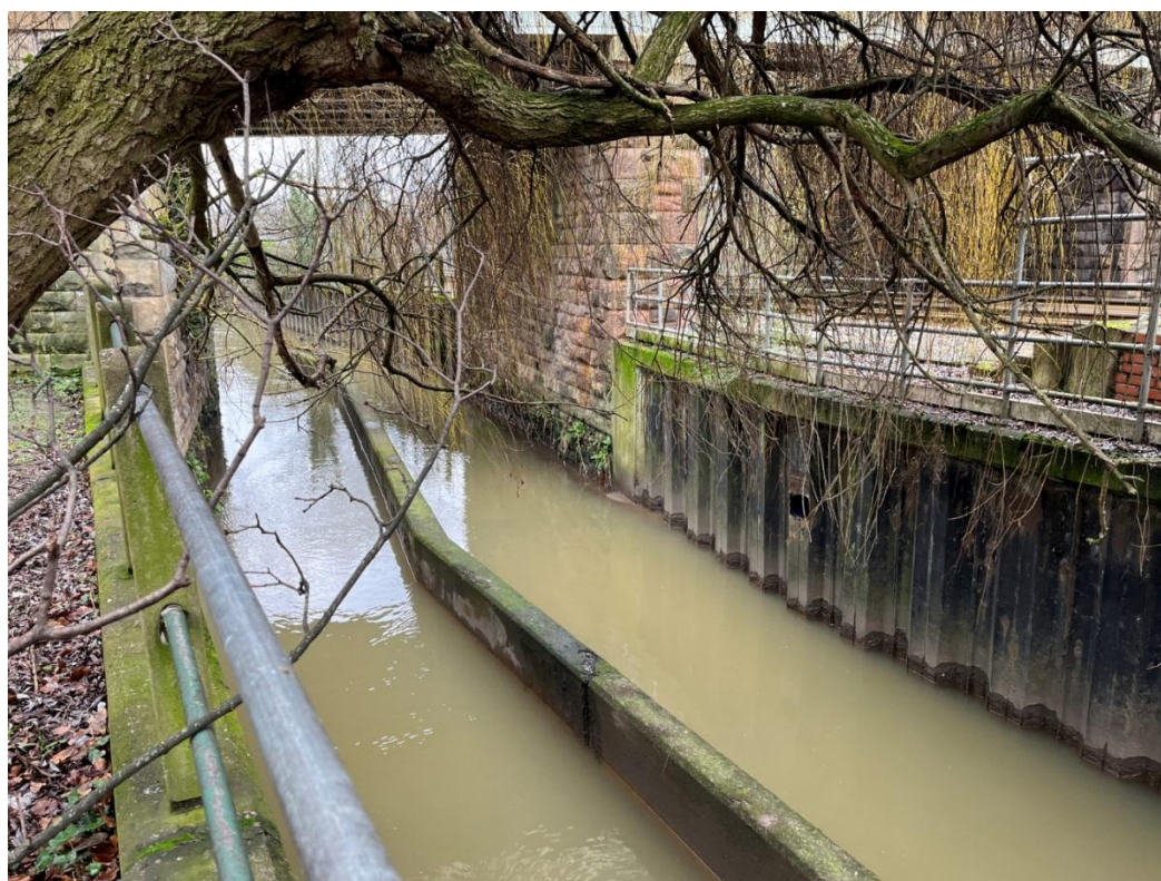
Figure 17: Another example of sheet piling on both RB and LB with a central maintenance channel divider at SK55342 42810. Section near St Leodegarius Church, Basford downstream of Church Street.
