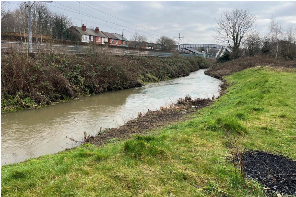
Figure 14: Lincoln Street Open Space. Widened area visible from Fig. 13, the confluence with the Day Brook enters under the tram lines from the LB. While care would be needed to avoid breaching the Sustainable Urban Drainage System (SUDS) ponds several metres outside the right hand edge of the frame, there may be opportunities to increase the degree of channel sinuosity and variation in width by altering and regrading the RB in this reach.
