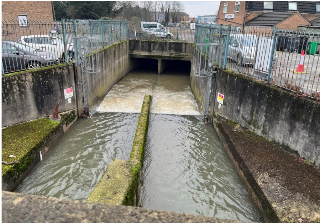
Figure 40: Very short, open section at SK54927 39200 with a weir and entering a further culvert (parallel to Hill Side). Structures photographed facing downstream while standing on the downstream end of the culvert cited for Fig. 39. Note the presence of a further, similar weir at the downstream exit of this culvert below the A6200/Derby Road at SK54932 39153.
