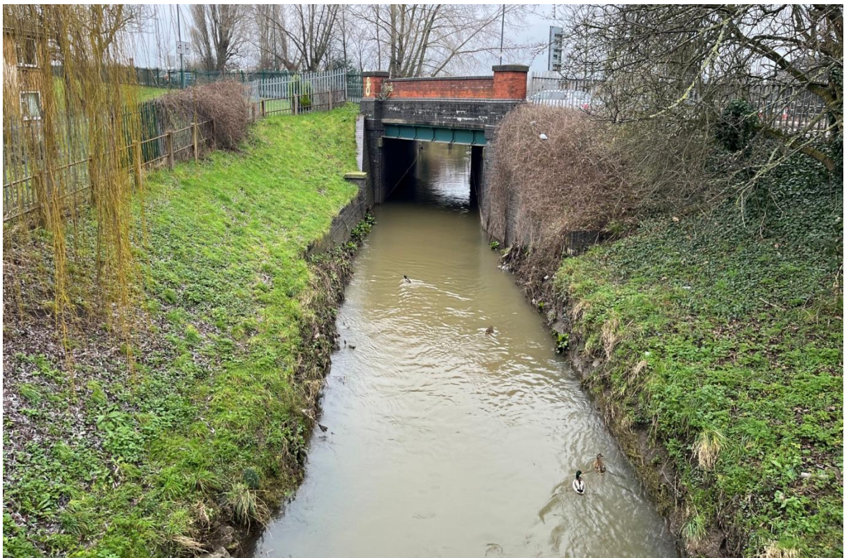
Figure 27: The channel adjacent to Poulter Close at SK5499641212 follows the typical design of straightened, artificial channel, flanked by grassed flood embankments (see also Figs 28 - 30).
