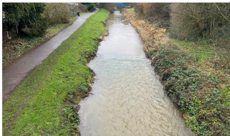
Figure 6: Upstream limit of the visit at SK54316 43872 (near Highbury Vale tram stop) straightened channel, small, submerged degrading weir.
