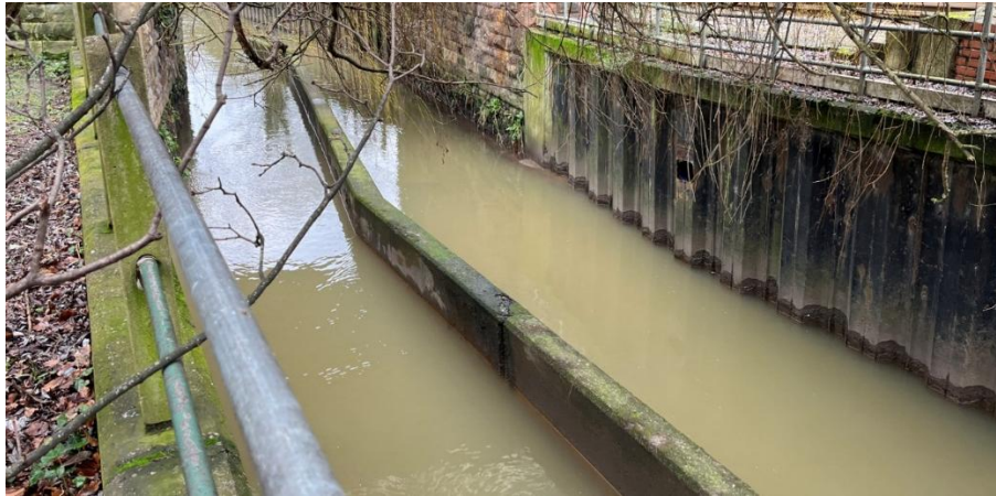
Figure 5: Central dividing wall for channel maintenance on the River Leen.
