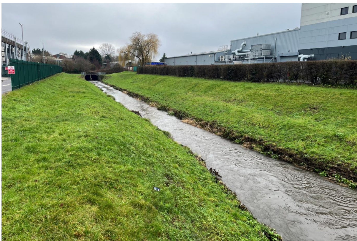
Figure 45: Below Willow Road Bridge at SK55488 38488 photographed from the LB within a formal flood defence channel. Any flooding resulting from the canal-crossing siphon appears likely to bypass these defences.
