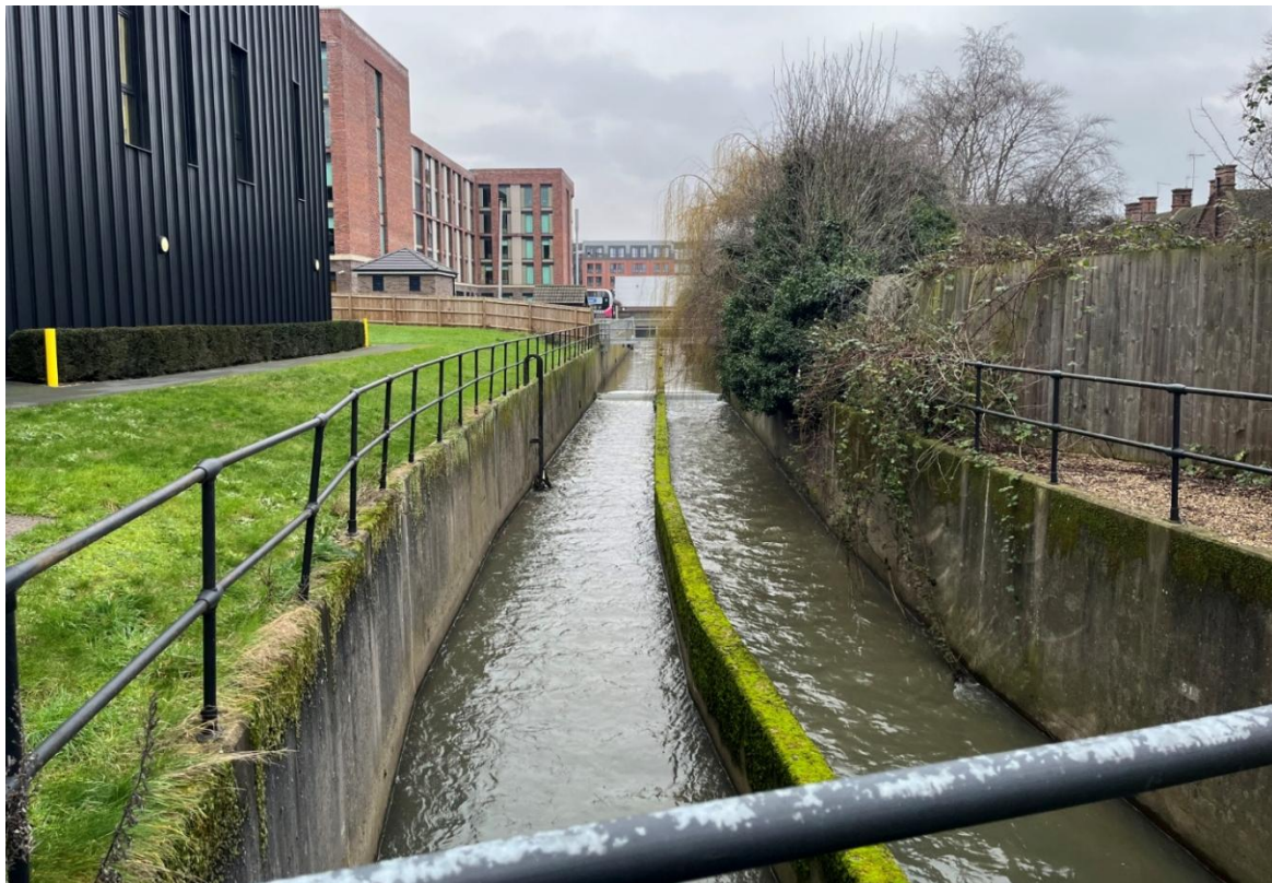
Figure 39: Standing on entrance to culvert facing upstream towards weir at adjacent to centre for aerospace manufacturing, University of Nottingham Jubilee Campus, SK54933 39242.
