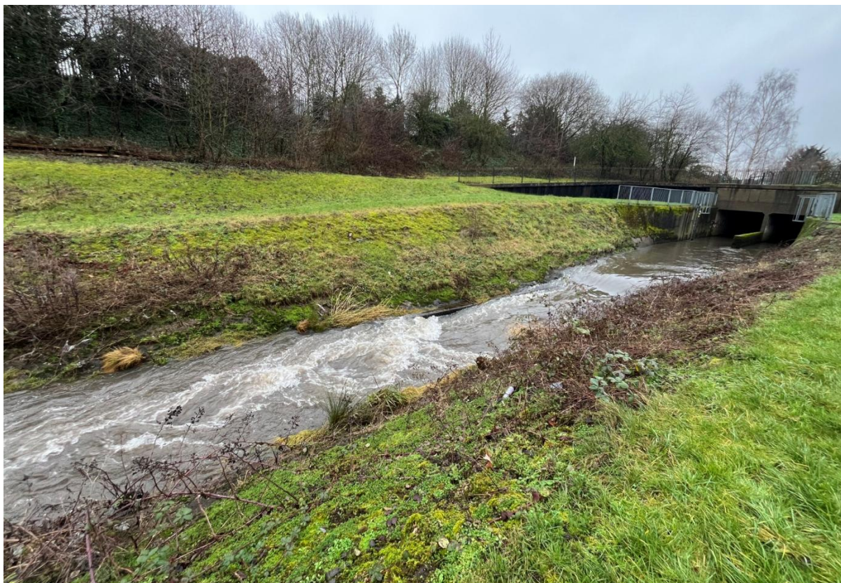
Figure 46: Weir downstream of Lenton Lane at SK55724 38374. Note hydraulic limit imposed by bridge.
