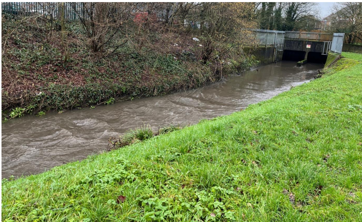
Figure 43: Emerging from Leen siphon (a structure with its own, implied flood-risk concerns) crossing under the Nottingham Beeston canal at SK55382 38600 with some slightly more structurally-diverse vegetation on the opposite bank.
