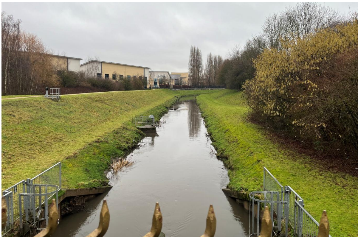
Figure 48: Facing downstream where the culvert cited in Fig. 47 ends at SK56001 38418. The Leen then enters another culvert 530m downstream of this point before its confluence with The River Trent at SK56647 38073, approximately an additional 270m downstream. This is the last open section of the Leen before it meets the River Trent.
