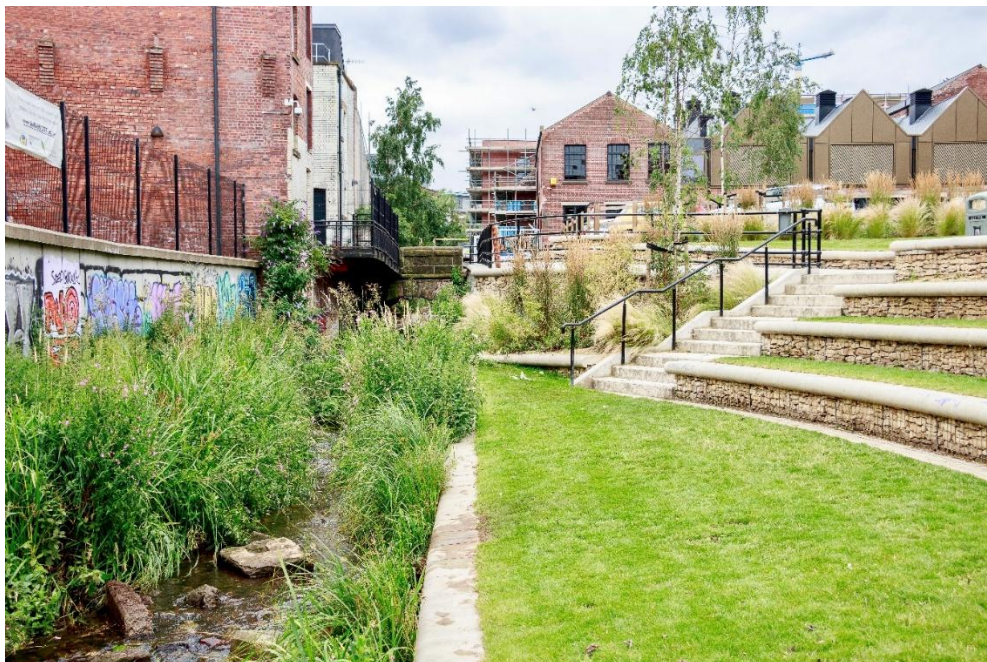
Figure 4: Facing upstream from within the previously-culverted channel and the pocket park. The black gantry attached to the white brick wall on the left (background) is visible in Fig.3 as the red gantry to the right of the frame in that image. In spate conditions, the river now spills over into the stepped amphitheatre.
