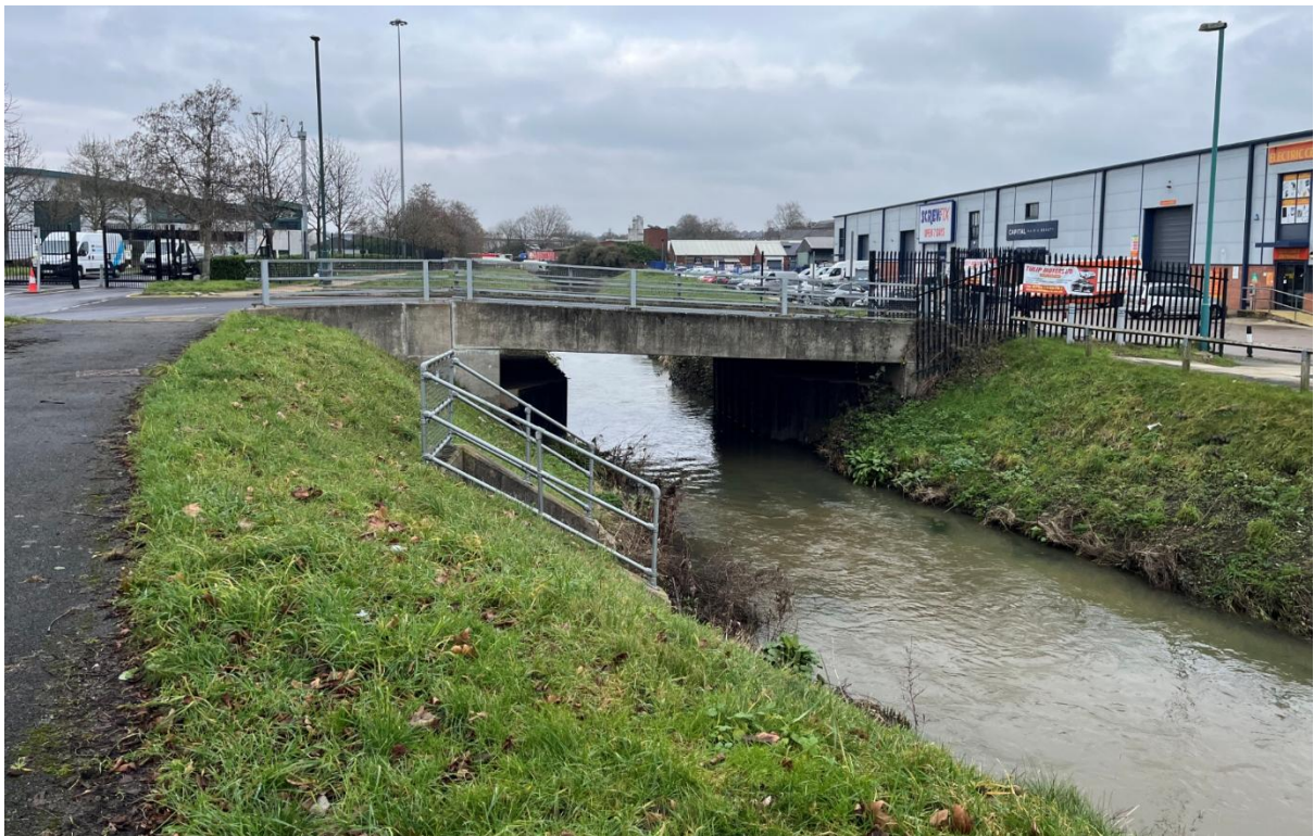
Figure 19: The hydraulic capacity of this bridge near the Wilkinson Street Tram interchange at SK55390 41999 is close to that of the bank-full height of the incised channel here. Being surrounded on all sides by transport and industrial infrastructure leaves little room for alterations to the channel form.
