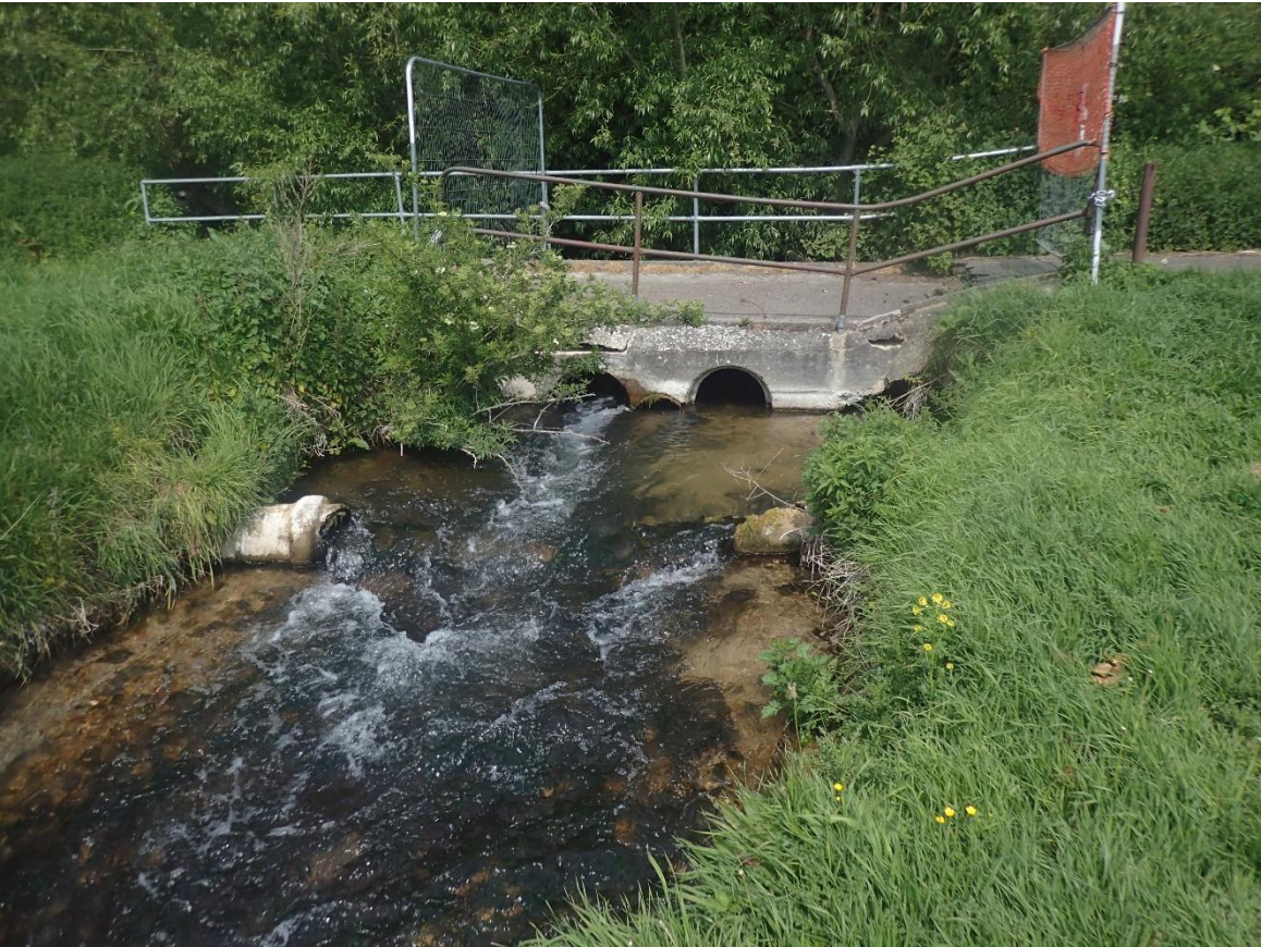
Photo 15 The collapsed culverted bridge as the watercourse turns back toward the old Kennet. This becomes a fast, high gradient section of watercourse down to the Kennet confluence, with space to regrade banks and re-meander the stream.
