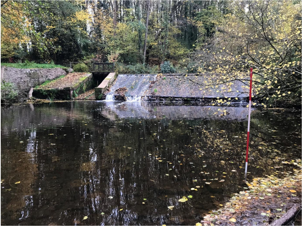
Photo 5 (52.165956 , -2.3690000) The large weir on the reserve. This structure currently severs the watercourse making it impossible for fish to move up and downstream when they need to. It also prevents the natural downstream movement of coarse riverbed material required to shape the channel and build habitat (Figure 2). The weir is in place to feed a historic corn mill leat, now used for an ornamental pond in the property on the RHB. This structure has been reviewed previously, and several options would be possible to mitigate this barrier in the river. This weir is a likely cause of the exposed bedrock in the channel downstream and lack of depositional areas of coarse sediments creating channel, flow and habitat diversity (impacting geomorphological process – Figure 3).
