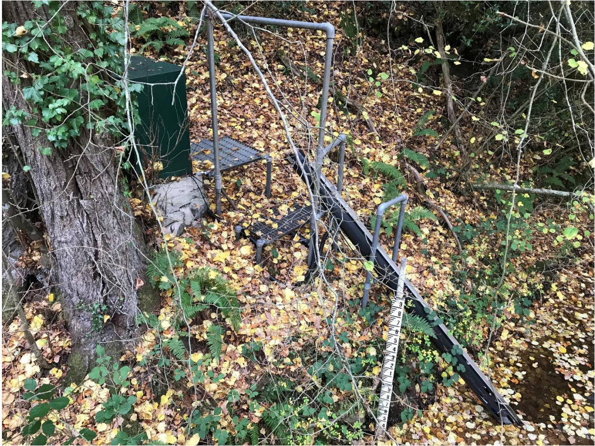
Photo 23 (52.159993 , -2.3740597 ) A river level gauging station was discovered at the upstream end of the reserve. This is owned by the University of Worcester; an absolute asset for monitoring conditions experienced by aquatic wildlife in the brook and should be brought back into action!
