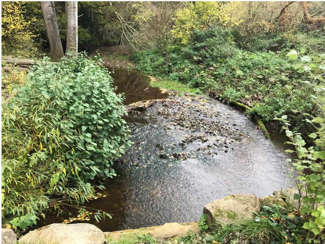
Photo 10 Looking upstream from the Pack Horse Bridge where flowing water returns, along with a riffle. It is possible this has formed due to the presence of the bridge slowing flow and causing deposition of material here.
