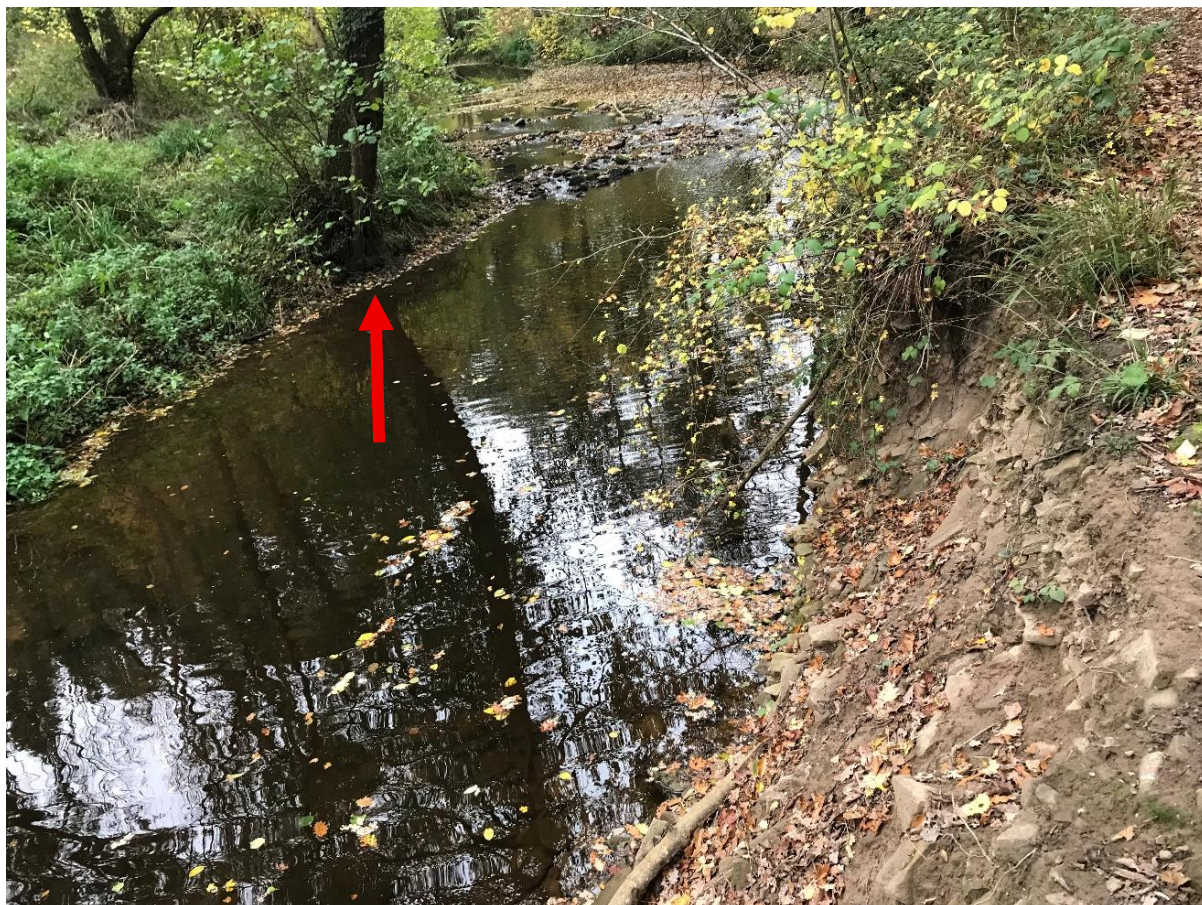
Photo 20 The first tree immediately upstream of the erosion on the RHB (red arrow). A great location right by the channel and potential to fell across the river or use the stump as an anchor for a tree kicker.
