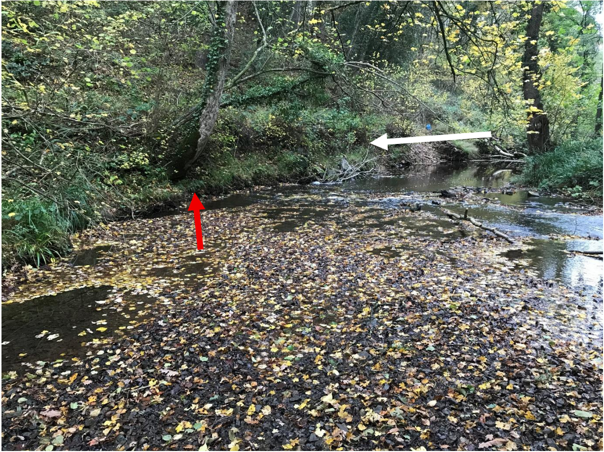
Photo 21 The next two trees upstream, perhaps using the stem on the true right bank (red arrow) as a kicker the large tree on the true left bank felled over the channel in the direction of the white arrow.
