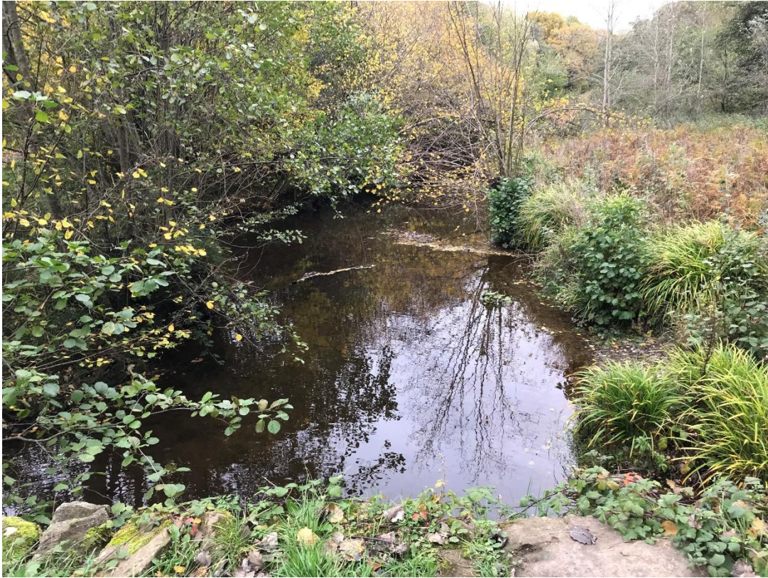
Photo 9 (52.163835 , -2.3684206) The Pack Horse Bridge looking d/s into the start of the impounded section caused by the weir, 270m downstream.
