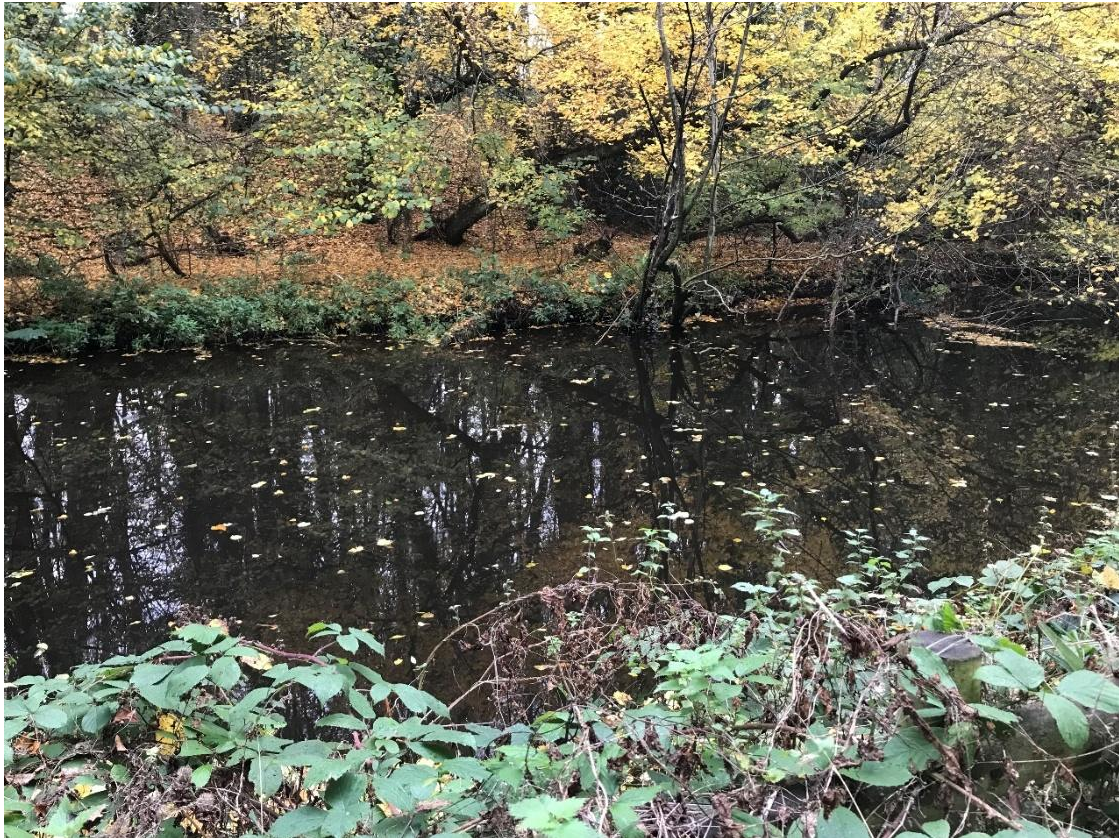
Photo 7 (52.165078 , -2.3687537) Water is impounded for a long distance upstream of the weir (>250m) due to its size relative to the watercourse, creating pond-like conditions where there would be stream habitat naturally!
