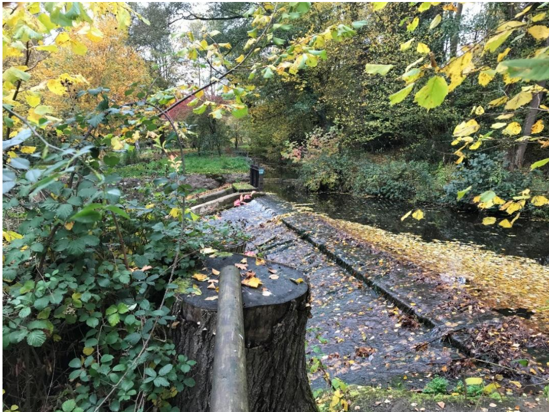
Photo 6 The impounding effect of the weir, forcing water into the old mill leat behind (just upstream of the sluice on the far bank in this picture).
