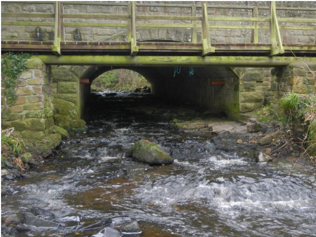
Photo DSCN6364. Being clear-span and located on bedrock, the A69 road bridge poses no significant additional issue for fish passage into the burn. As with many of the Tyne tributaries, it is naturally challenging.
