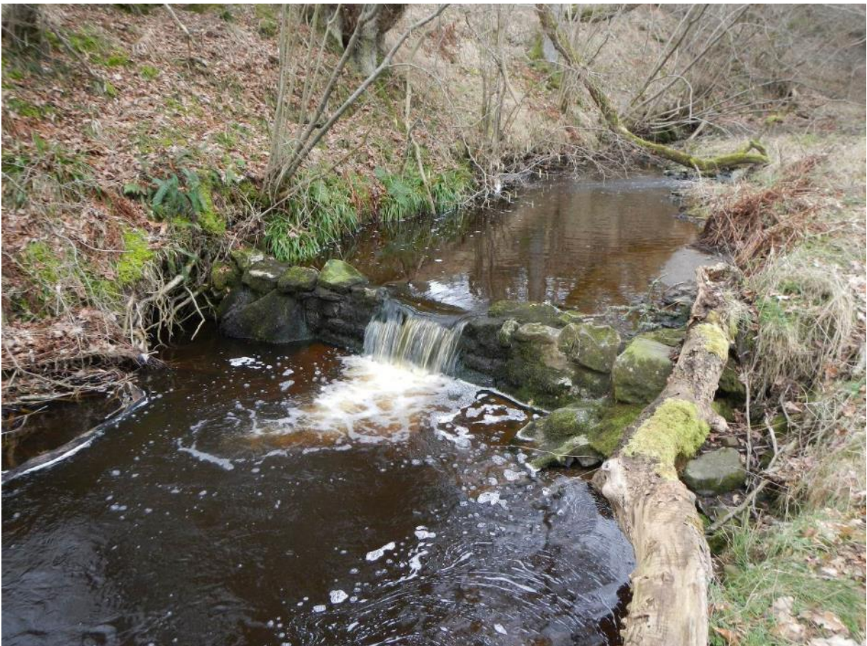
Photo DSCN. A small weir within Tony's Patch Nature Reserve (NY 82239 65641) poses an unnecessary and significant obstacle to fish passage. A small structure like this could be easily removed by a group of volunteers, to reinstate habitat quality and connectivity.
