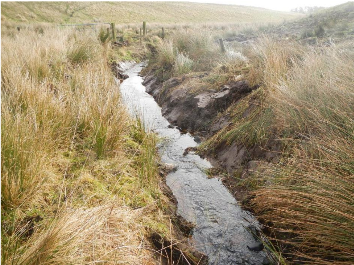
Photo DSCN6178. From NY 81914 67483 - NY 82443 66994, major recent dredging has been undertaken, greatly degrading the channel and liberating large volumes of fine sediment into the burn.
