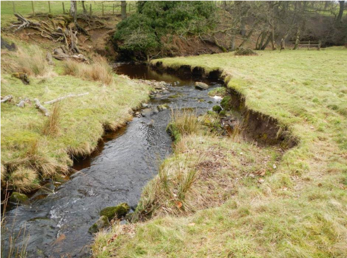
Photo DSCN6303. Grazing is undertaken in the two fields between the nature reserve wood and the next road crossing d/s (NY 82222 65425 – NY 82290 64956). Correspondingly, the riparian habitat quality decreases and bank erosion increases.
