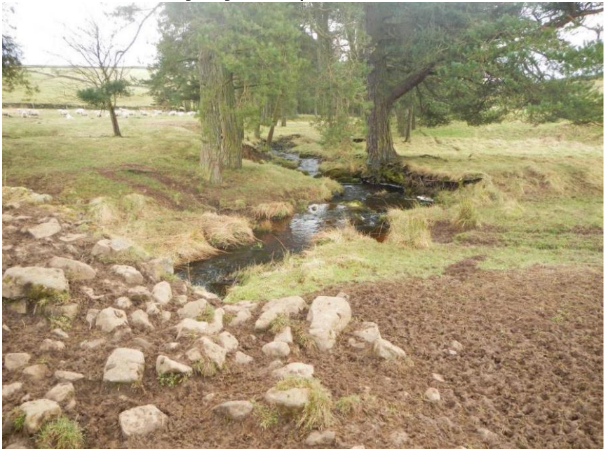
Photo DSCN6226. Although historically straightened d/s of the lonning, the channel is recovering some of its natural sinuosity, with bankside trees improving its diversity, despite being only a short distance u/s of a now defunct dam that would have originally impounded flows. Grazing also resumes d/s of the lonning.
