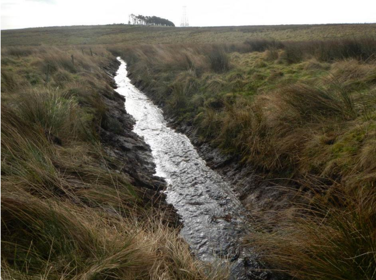
Photo DSCN6192. Further dredging of the straight channel denudes habitat and creates more fine sediment input that will impact upon habitats d/s.
