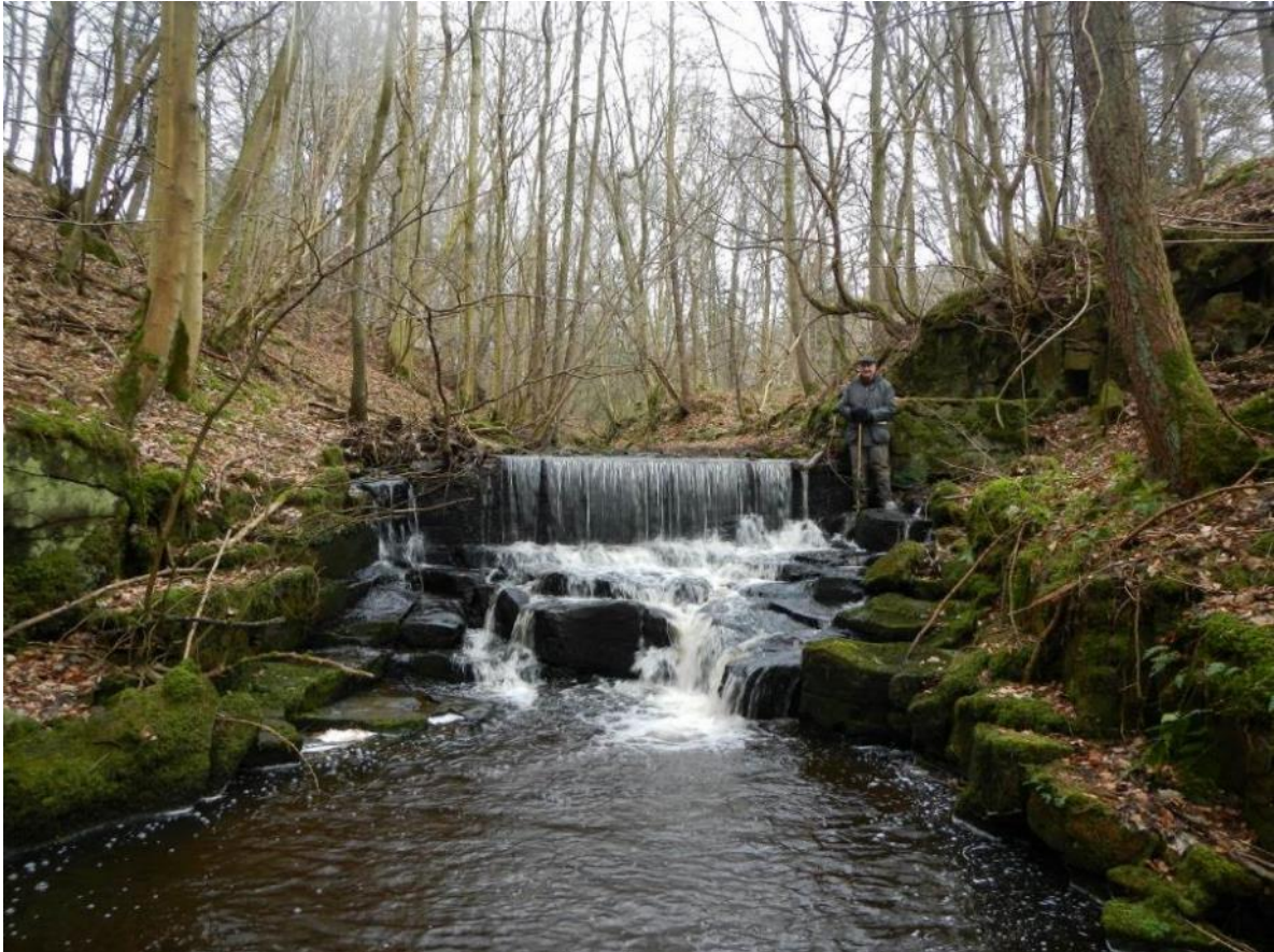
Photo DSCN6339. Further d/s, the valley becomes steeper and bedrocky. A stone weir built on top of a natural bedrock outcrop to supply a water wheel creates an impassable barrier in most flows (NY 81959 64846). This could easily be removed to return fish passability at the site to a natural state.
