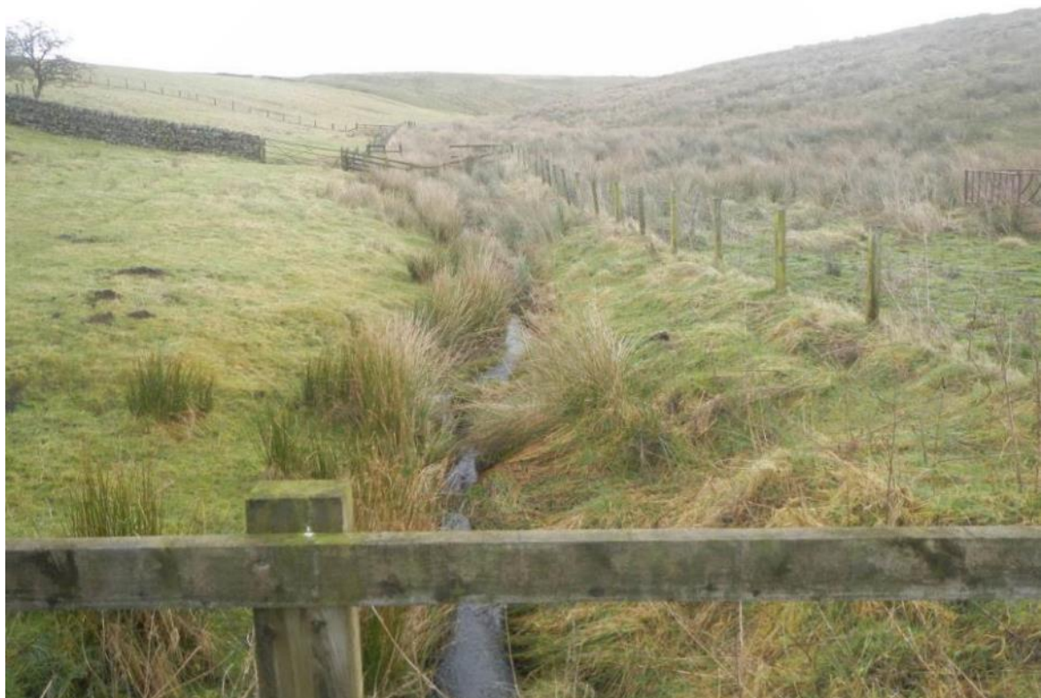
Photo DSCN6172. Looking d/s from the u/s limit. From this point d/s, the valley characteristics suggest there would have been a more defined watercourse here originally, but straightening and dredging have clearly been undertaken historically.
