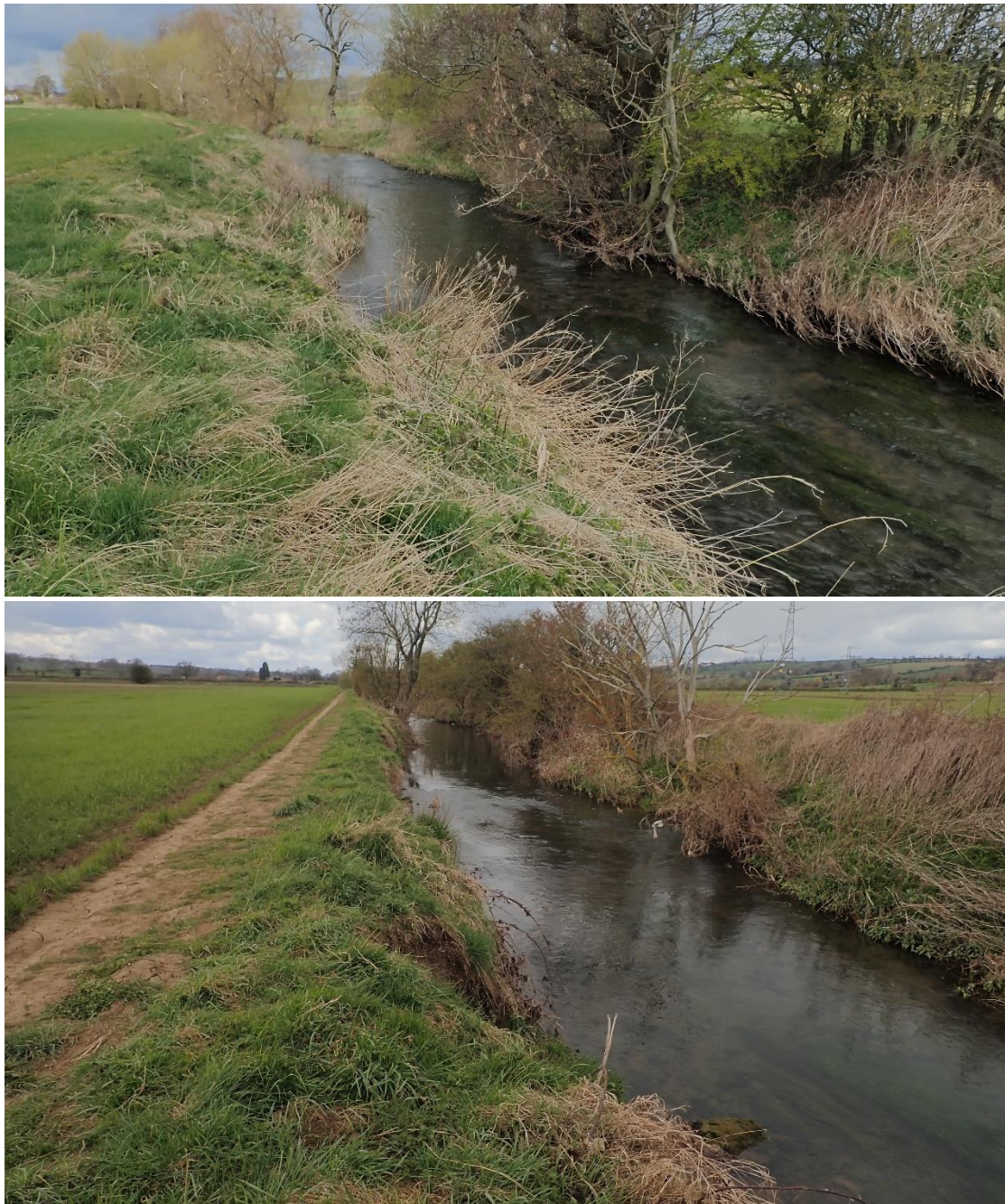
Fig 7. Straightened sections with a reasonably natural and ample 'buffer' zone from the intensive agriculture on the LB. Less cover and space was given on the RB, although it was appreciated that the native grass and herb cover would grow to >1m. More troublesome was the proximity of the field boundary squashing the footpath to the very top of the RB. There was notable erosion of the RB exacerbated by the compaction of the bank and the lack of buffer.
