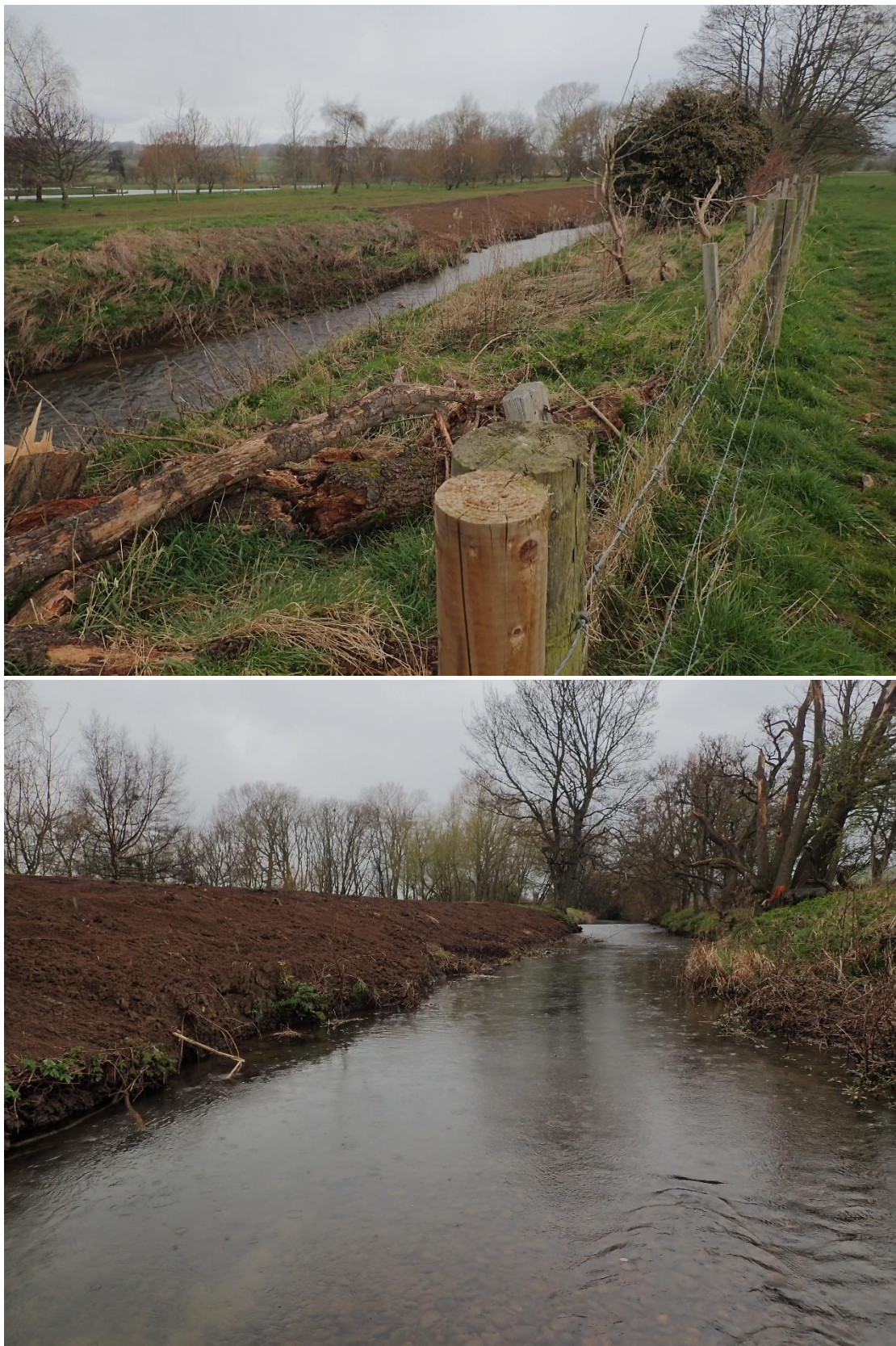
Fig 10. At NZ 17770 05360, the d/s limit of the upper beat, the landowner on the RB had taken it upon themselves to reprofile ~120m of bank and remove all the trees, plus remove low cover from the LB. There was no evidence of mitigation procedures to trap fine sediment which was smothering the entire bed, and this was probably unsanctioned work. North Yorkshire County Council would be the relevant authority.
