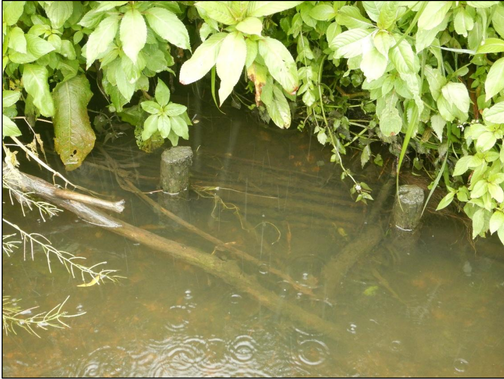
Pic 5 – Some installed faggot bundles in the brook have not entrained fine sediment, and now the wood has degraded a void is left. Where posts can be found, they could be used to hold more wood gathered from nearby shrubs. The silt was probably flushed out due to shading from tall vegetation above, with shade the root structure is weakened. See example of brash and timber fixing in Recommendations.
