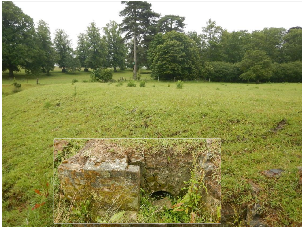
Pic 33 – A defunct sluice off-take from the river was found. It was later stated that it once directed flow to fish rearing ponds when levels in the channel were kept higher. It serves no purpose now but is an interesting reminder of how this chalkstream once had enough water to push flow in multiple directions for a range of purposes. It should be retained for its historical interest.
