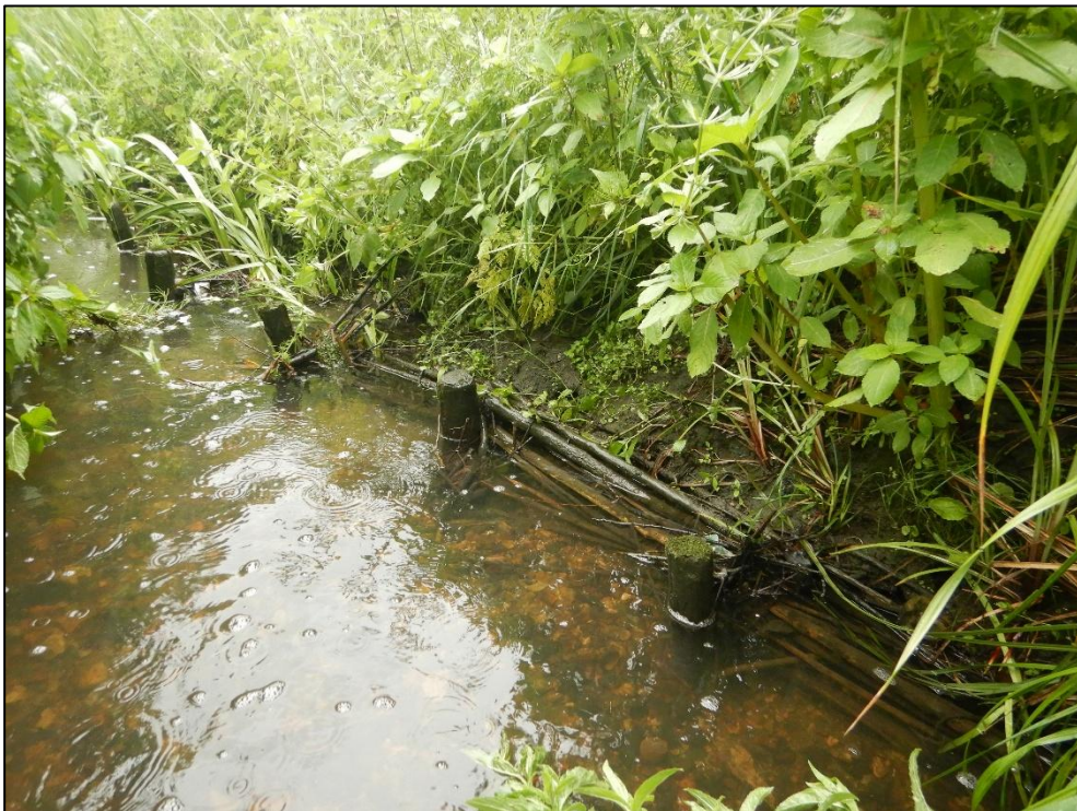
Pic 6 – Some faggot edging has retained fine sediment and provides a rooting substrate for marginal vegetation along the brook. Control of the invasive non-native species, Himalayan balsam, would aid the growth of native plants beneficial to marginal vegetation development. See example of invasive plant species control in Recommendations.
