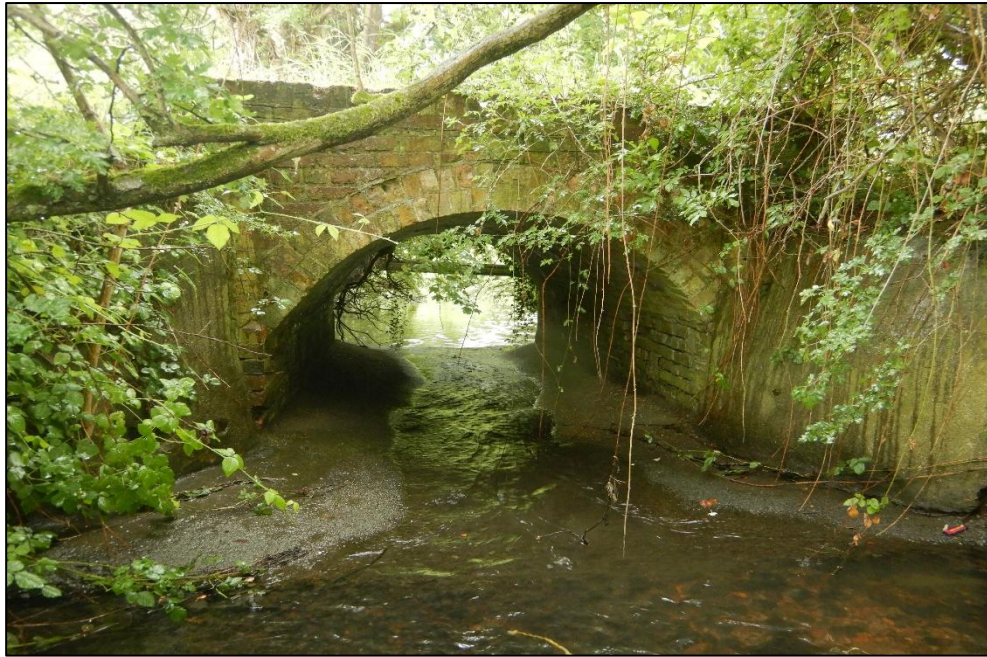
Pic 13 – The same bridge as Pic 12. Given that this bridge is a short distance from the last, and that it had not been accessed for recent meadow management (suggesting concern for its strength), the best option in terms of river restoration would be to remove the bridge. The bridge is causing an impoundment, and with its removal, flow diversity would be restored to the upstream channel, with the potential to mobilise important bed substrates that will aid natural channel processes downstream (such as riffle formation). The upstream channel may even start to naturally meander. The best outcome would be to package the bridge's removal with channel realignment. The bridge impoundment presents similar problems that weirs cause to rivers, see bridge removal in Recommendations.
