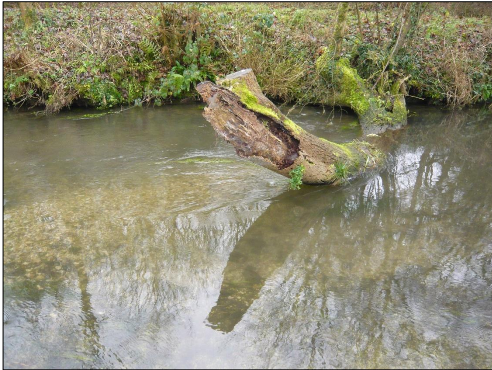
Pic 50 – Timber positioned above the bed can enhance bed scour, a useful approach in low energy chalkstreams.
