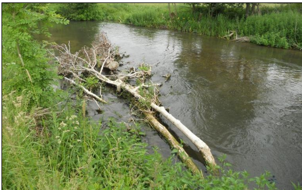
Pic 45 – Pining of LWM in margins for cover, sediment accretion and flow deflection. The complex cover provides excellent protection for trout fry.
