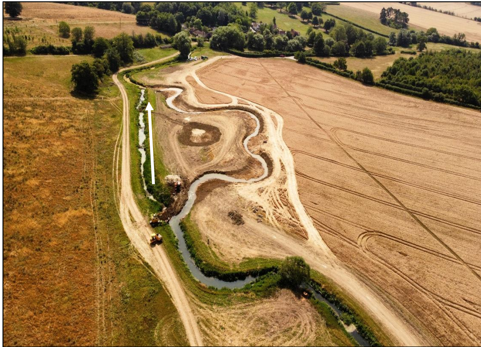
Pic 53 - Channel realignment to create a new longer sinuous channel where it previously ran in a straightened channel (white arrow).
