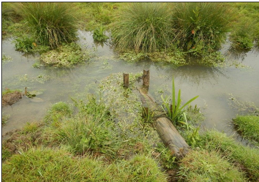
Pic 34 – A flow deflector in the cattle poached reach. It had no effect, mainly due to the constant disturbance caused by cattle and secondly due to the limited gradient of the reach reducing the river's capacity to drive flow against the bed to create scour. It would be more effective to install large tree trunks across the river at differing heights to make use of high flows. If needed gentle excavation of the bed beneath such structures could be done to initiate bed scour.
