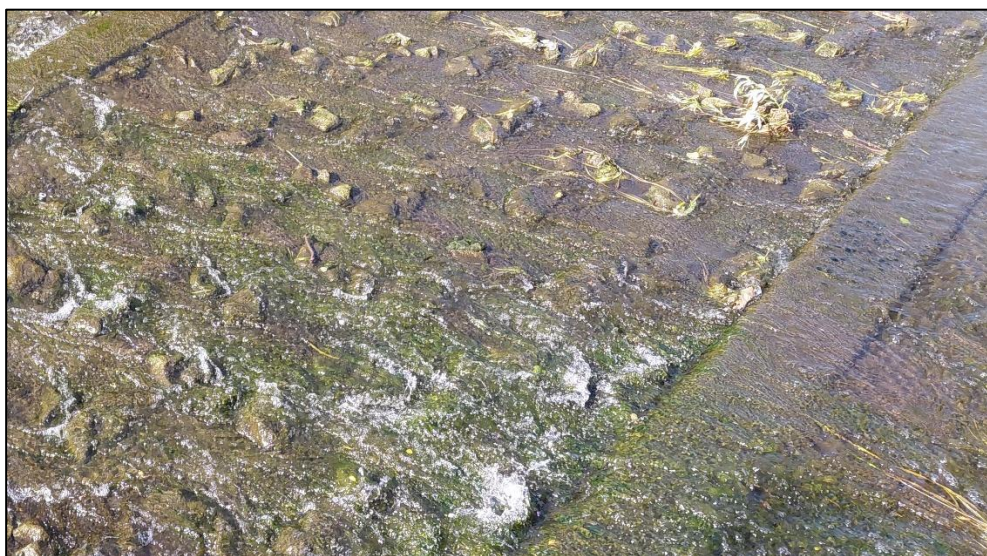
Pic 54 – Stone sets to increase channel roughness to aid fish passage.
