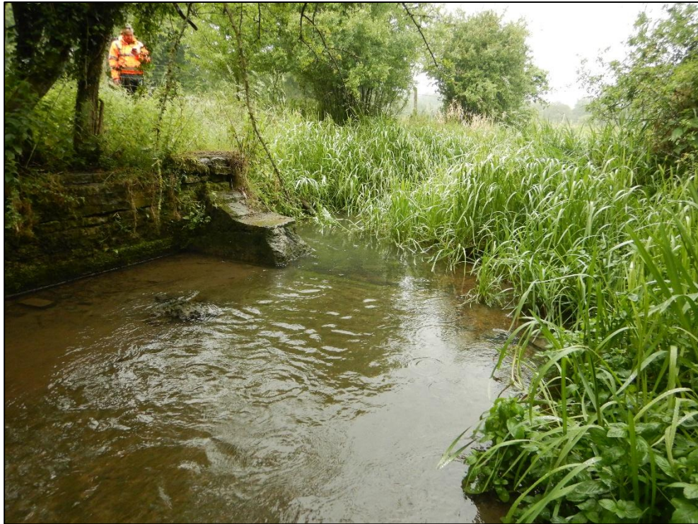
Pic 17 – The base of a former weir has been retained after its partial removal. The effort to remove the barrier is commended but the issue is not resolved until the concrete base of the structure is removed. With ~4m of concrete base in place, downstream sediment transport is interrupted, an impoundment is created and fish passage in low water is not as good as it should be.
