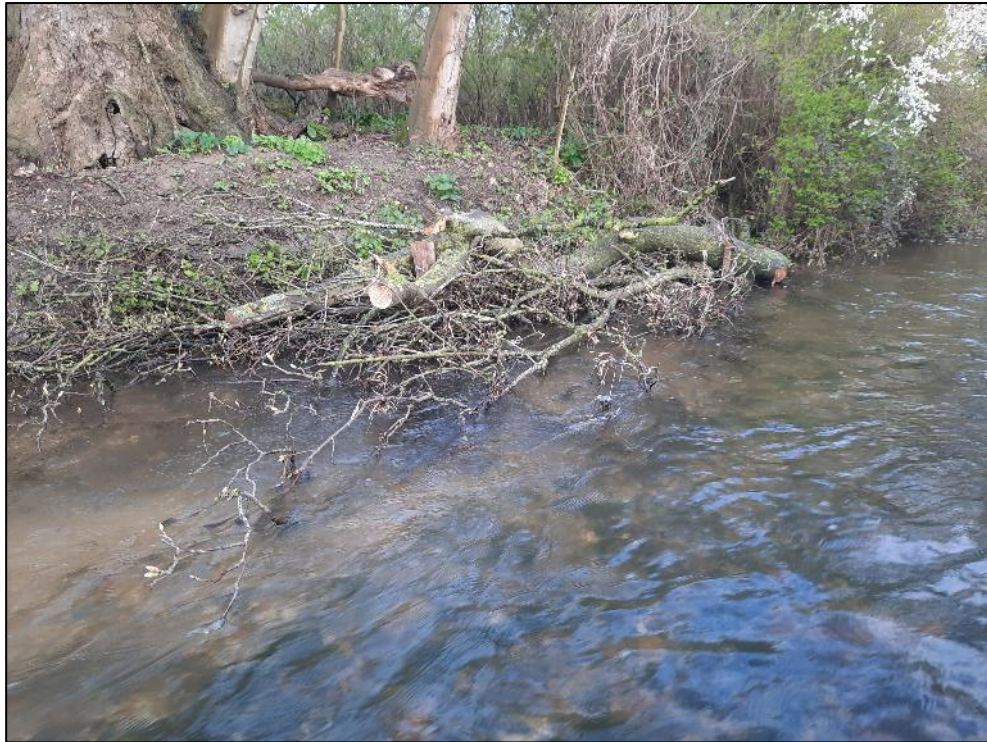
Pic 48 – A more structured (and secured) approach sees the construction of a brash ledge. This has brash and timbers layered to hold the smallest pieces below water. Chestnut posts and steel wire is used to secure the material. This type of feature is good for sediment entrainment in depositional areas of rivers.
