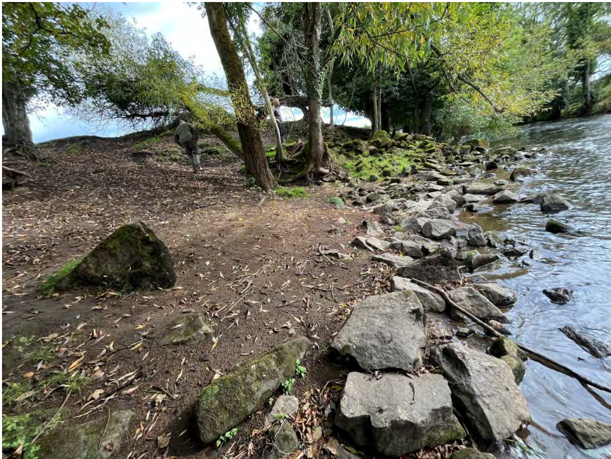
Figure 12: Collapsed (or deliberately positioned) stonework that appears to be used by stock as a watering point.
