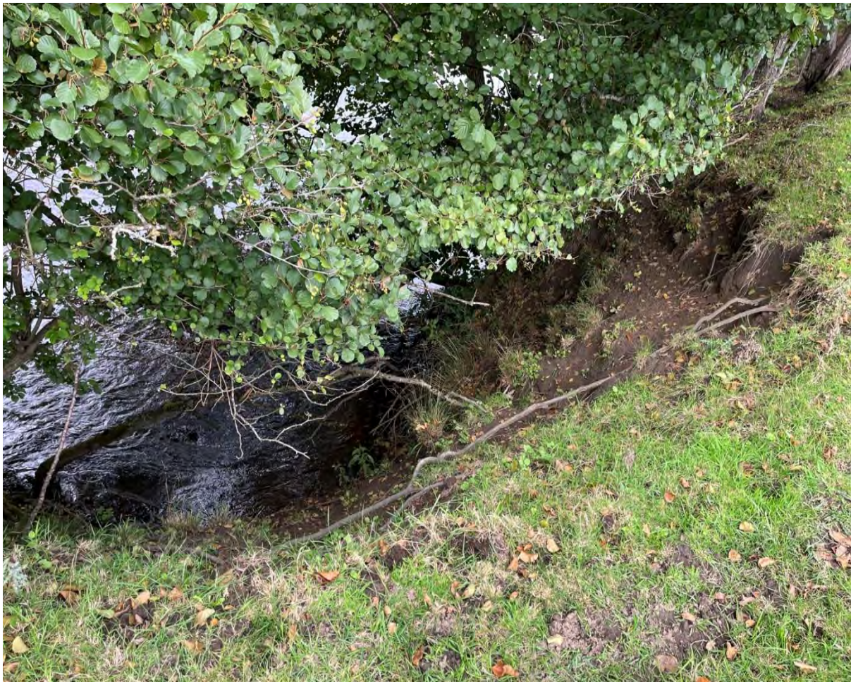
Figure 6: Steep, collapsed banking associated with trampling and the loss of deeper root structure created by over-grazing. Grazing intensity that is perfectly suitable for a farmers field is not suitable for a riverbank.
