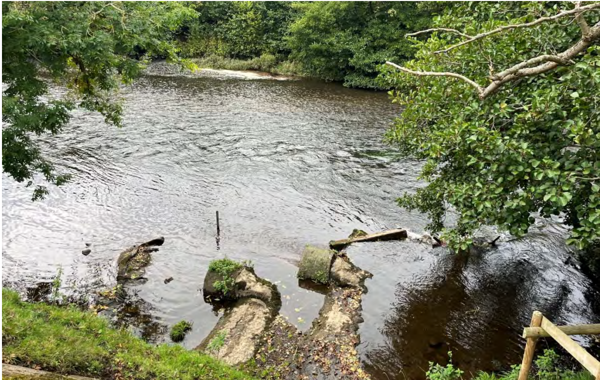
Figure 9: Dual pipes with their open ends facing downstream apparently associated with an old pumping station or other asset building at 53.170978, -1.612481.
