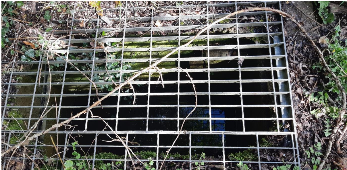
Figure 14: Looking down into chamber fed by the weir – with an apparently sealed connecting goyt – suggesting the weir may be redundant in terms of water diversion.
