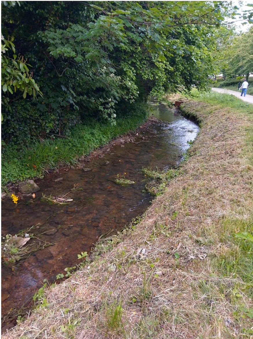
Photo 17 The Chelt along Honeybourne Way (51.903077 , -2.0873508). Straight and within a classic flood engineered trapezoidal channel shape. Due to lack of natural sediment supply, the substrate is mostly man-made materials but will possibly function with the same effect as larger cobbles and boulders found naturally in streams. Trout, bullheads and all aquatic invertebrates will use the structure as key habitat in this section. Leaf litter from the adjacent trees will provide basal resources for shredding and grazing aquatic invertebrate groups.
