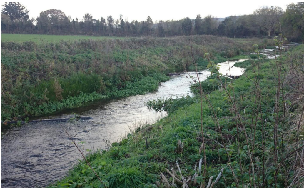
Figure 10 Regraded banks alongside modified channels allow natural river features and marginal plant growth to develop , without impacting flood water conveyance capacity. . In conjunction with a modelled suite of catchment wide flood resilience interventions, it may be possible to consider actions such as this on the Chelt, allowing nature to return at the same time.
