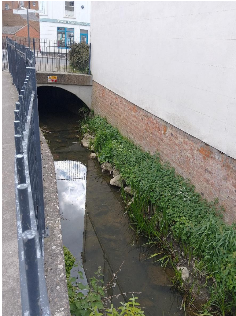
Photo 1 The start of the survey section by the Bayshill Pub. The Chelt resurfaces after several hundred metres of being buried under the town. The river is heavily modified, constrained by high artificial banks in a straight channel. The larger rubble in the bed will offer some physical habitat for fish and aquatic invertebrates, the accumulation of sediment on the left bank is allowing some vegetation to take hold. The emergent and trailing leaves provide a small amount of natural habitat structure as well.
