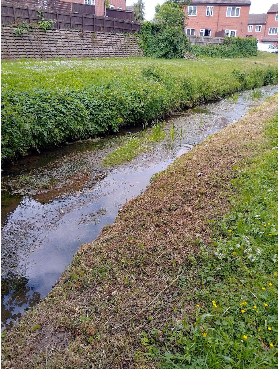
Photo 21 Removing a large amount of the bankside material here would increase flood water storage capacity, while also giving an opportunity to lower bank heights, re-meander the watercourse and create bed level diversity and
