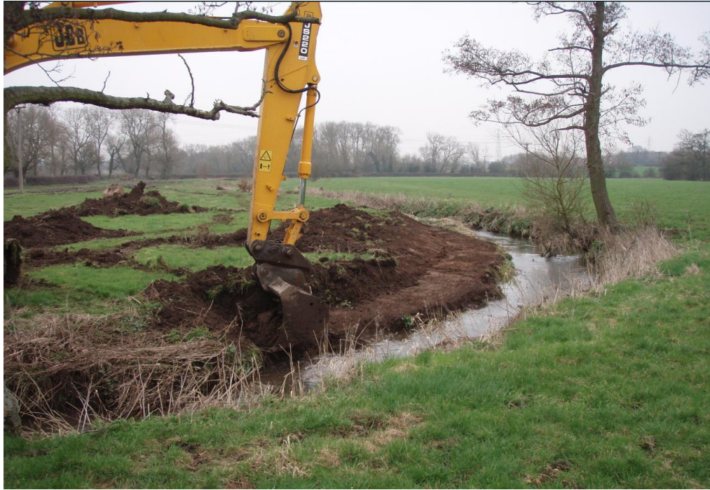
Figure 9 Pulling banks back will provide space for the water course and more flood water capacity, whilst easing impacts of high velocity flows.
