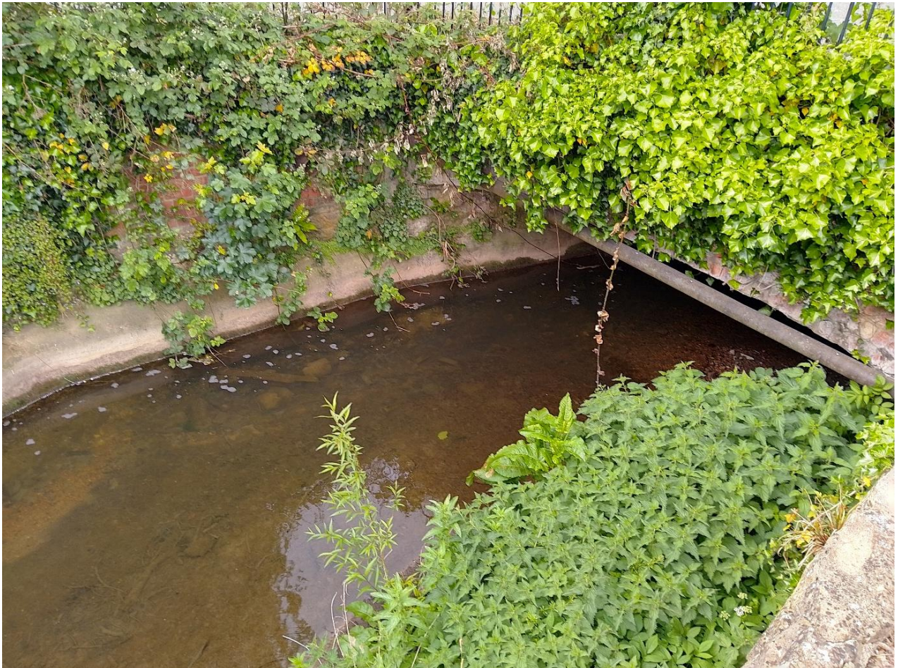
Photo 6 The culvert supporting the footpath onto Royal Wells Way (51.899522 , - 2.0816930).
