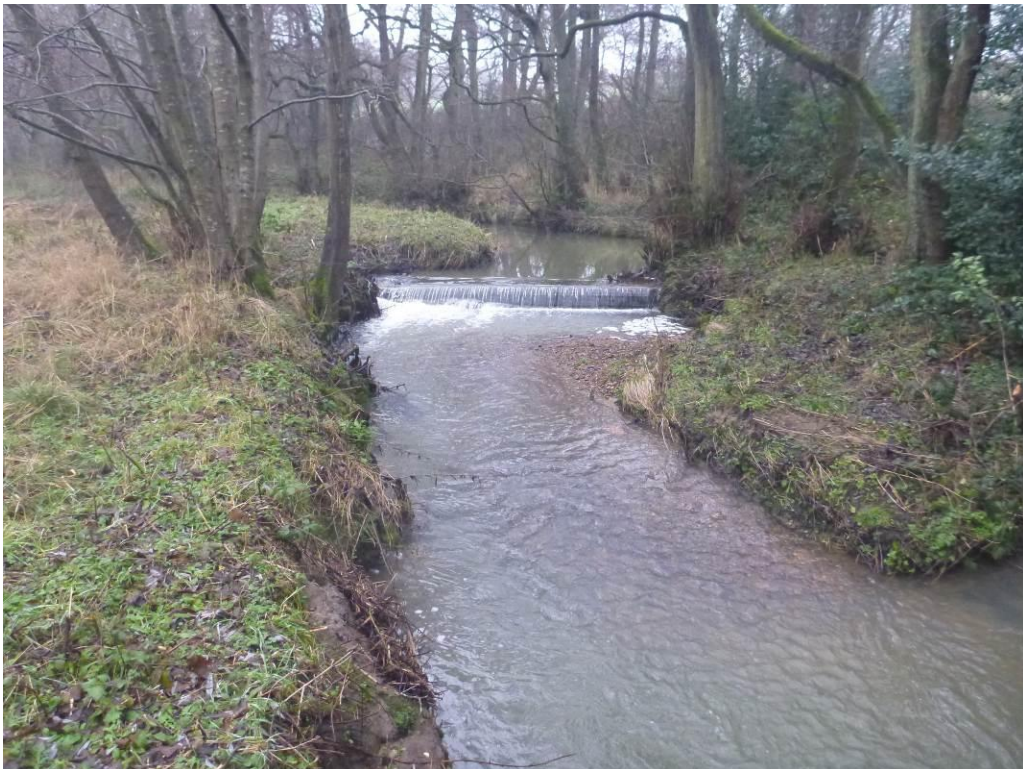
Photo 53 Typical weir within this section, constructed from hollow concrete beams.
