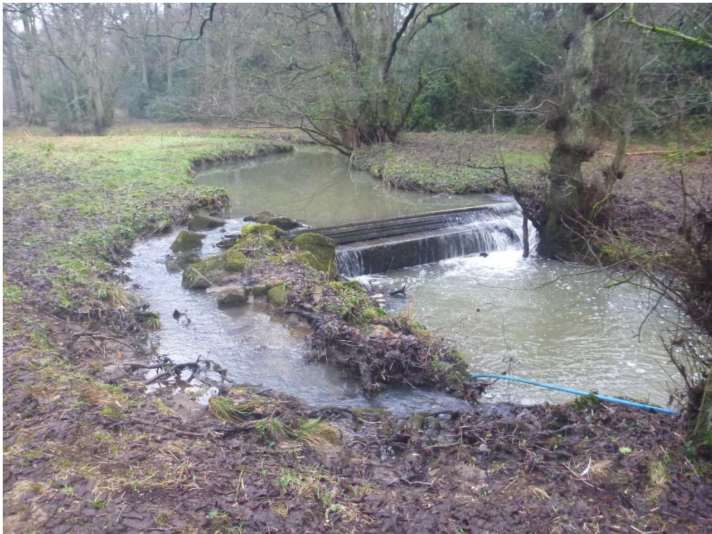
Photo 61 Weir in Figure 1 B
