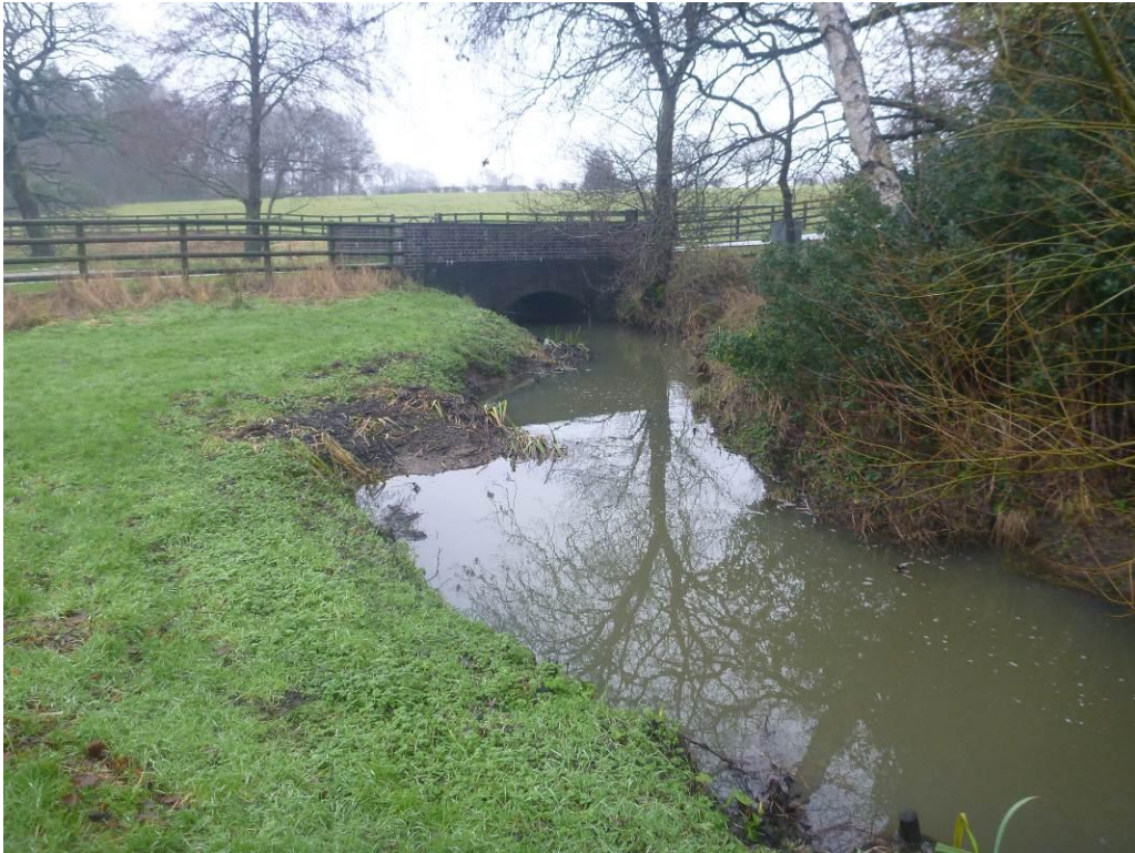
Photo 32 Impounded reach above weirs in Photo 31 towards Blue Bridge.
