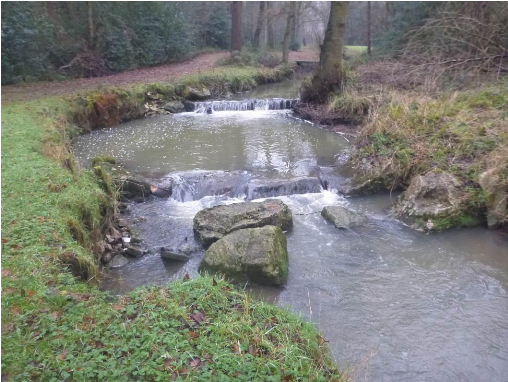
Photo 36 (52.991435, -1.635491) A retained weir and subsequently constructed boulder pre-barrage (foreground), and the same area in 2015 below.
