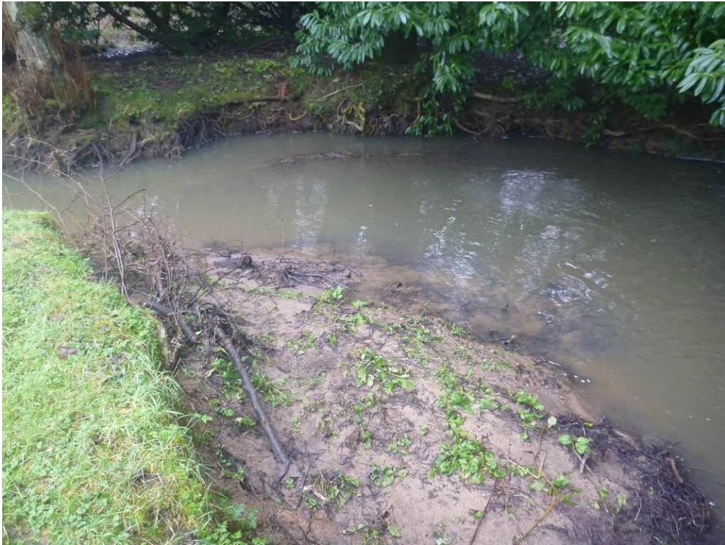
Photo 24 Deposition of fine sediment within a brushwood mattress on the inside of the bend in Photo 25. This, along with the turbid water, highlights an issue with fine sediment inputs further upstream.
