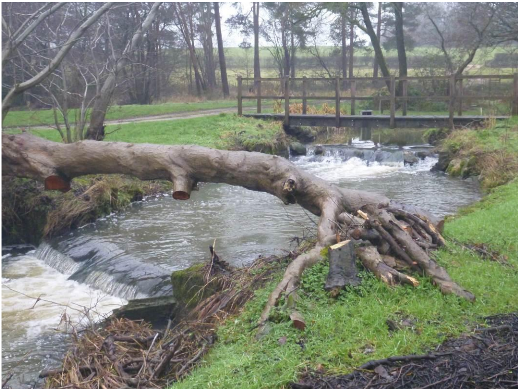
Photo 19 Weirs leading up to hatchery ponds offtake
