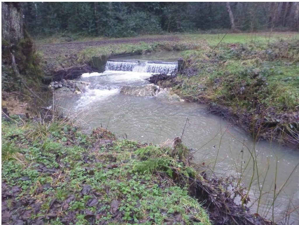
Photo 43 (52.992460, -1.635787) Notched weir and pre-barrage, and same structure below in 2015 (Photo 44).
