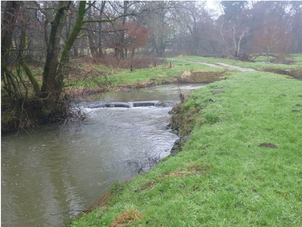
Photo 16 Weir upstream of Photo 15
