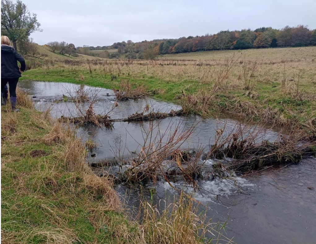
Photo 13 Example of the use of living willow ‘weirs’ to stabilise introduced bed substrate at the transition in levels between a restored river/floodplain (upstream) into the incised, historically modified channel downstream (upper River Witham, Lincolnshire).
