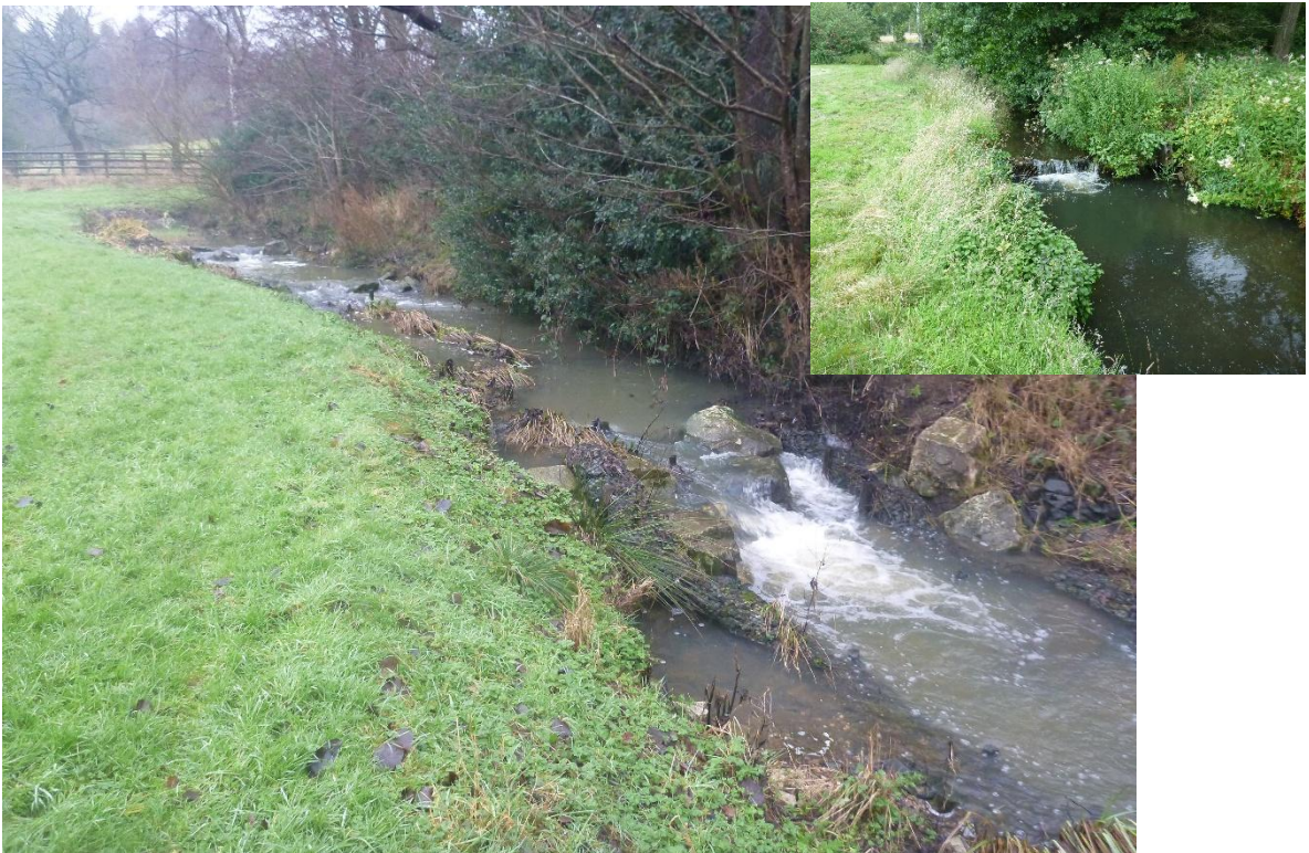
Photo 31 Boulder weirs and the type of structure they replaced (inset).
