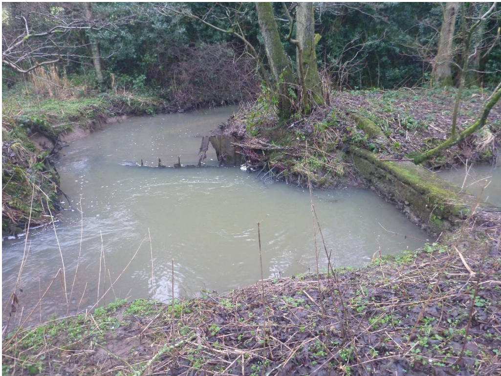
Photo 63 (53.001672, -1.6333821) Channel bifurcation with weir (right) and remains of sheet piling (left).
