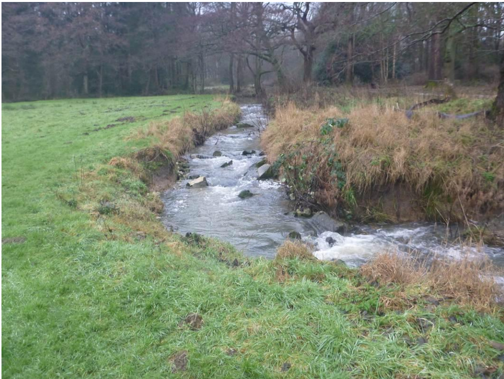
Photo 27 Rock ramp maintaining water levels for the Sandy's Lake offtake.
