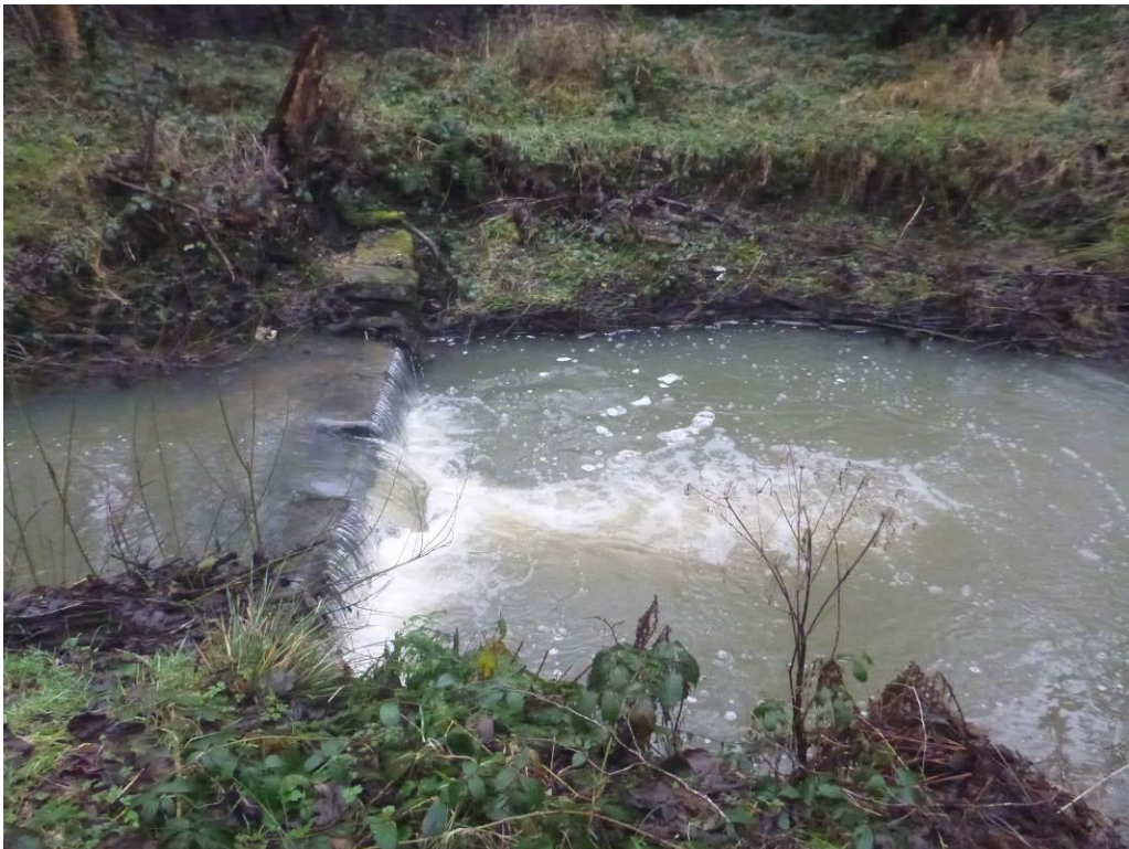
Photo 41 (52.992452, -1.635620) Notched weir and same structure below in 2015 (Photo 42).
