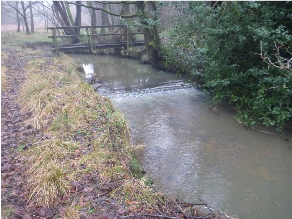
Photo 52 Public footpath bridge and one of numerous weirs.
