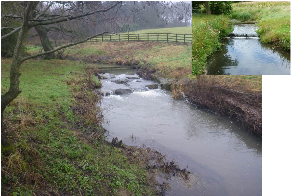
Photo 33 (52.989597,-1.6358706) Boulder weir immediately upstream of Blue Bridge, and structure it replaced (inset).
