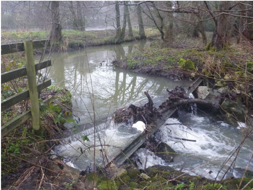
Photo 58 Weir in Figure 1 E
