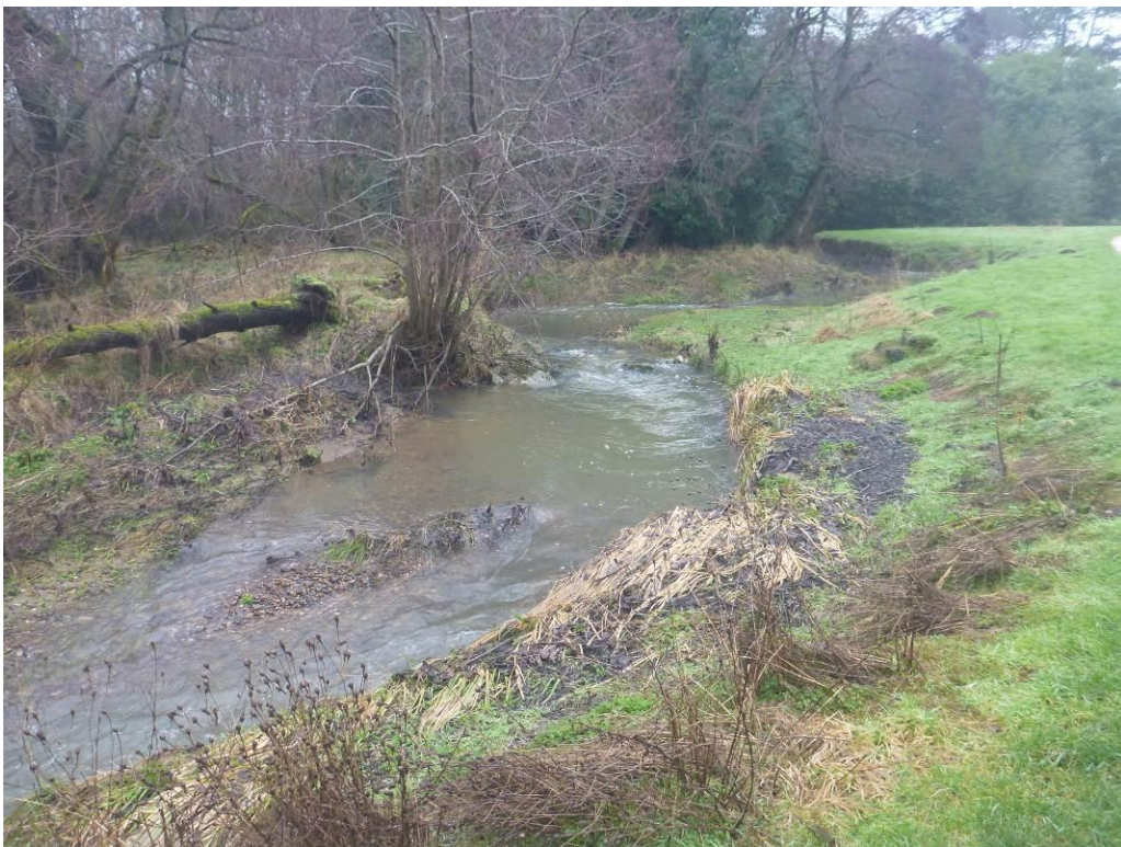
Photo 23 Weir removal and left bank reprofiling (right of shot) have greatly improved this area, leading to development of gravel features. Note the improved morphology where the channel has greater sinuosity and more varied dimensions.
