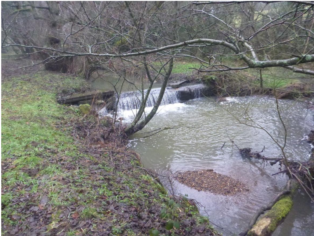
Photo 60 Weir in Figure 1 C
