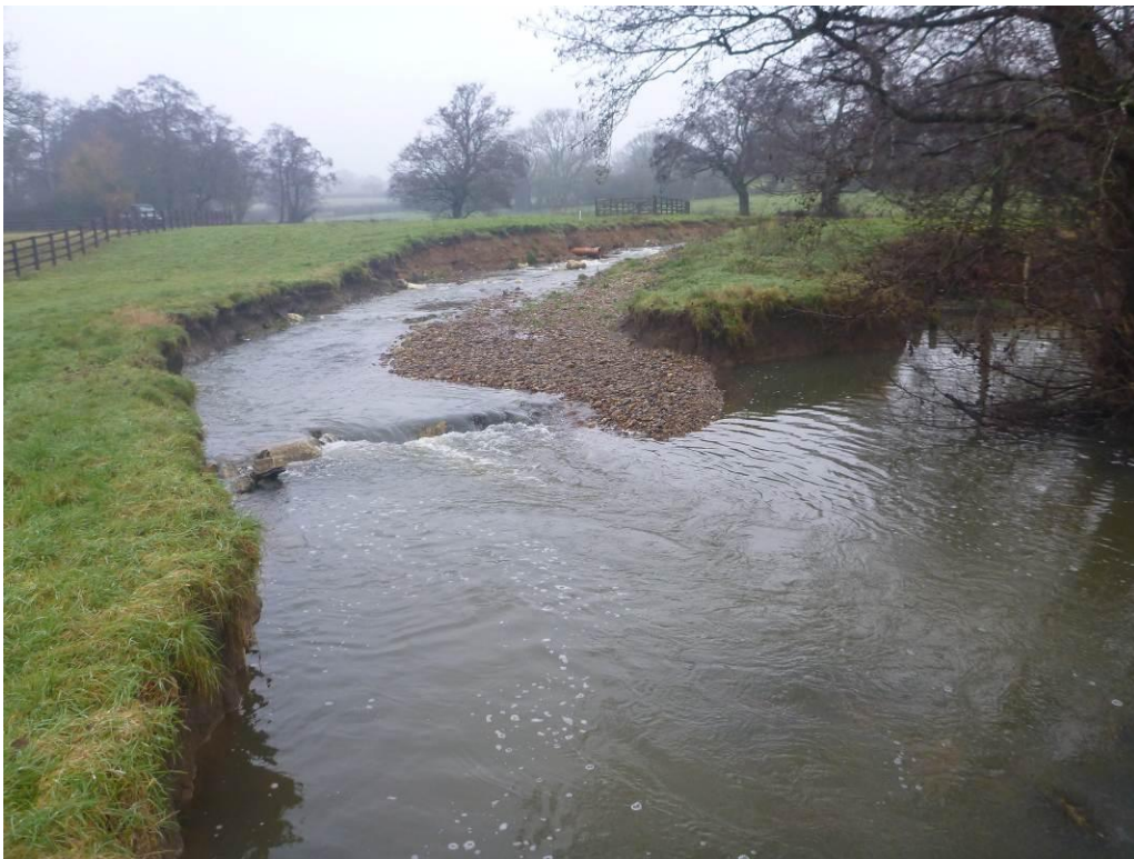
Photo 11 Rock ramp and former leat overflow channel (right), now a backwater.
