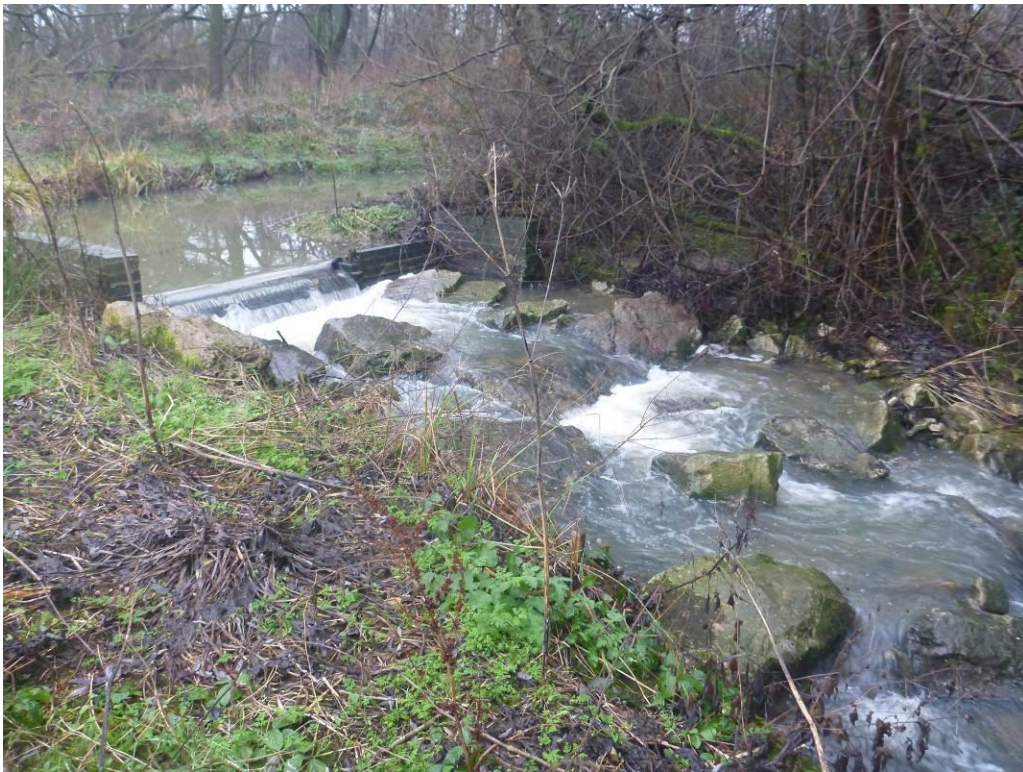
Photo 49 (52.994224, -1.635426) Rock ramp installed downstream of the weir maintaining water levels for Secret Lake offtake.
