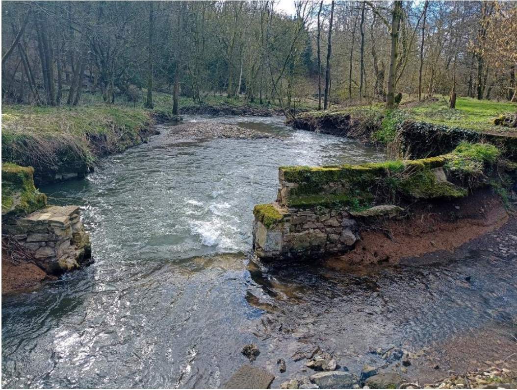
Figure 26 Notched weir (downstream view). Note freshly deposited coarse sediment on mid-channel bar.
