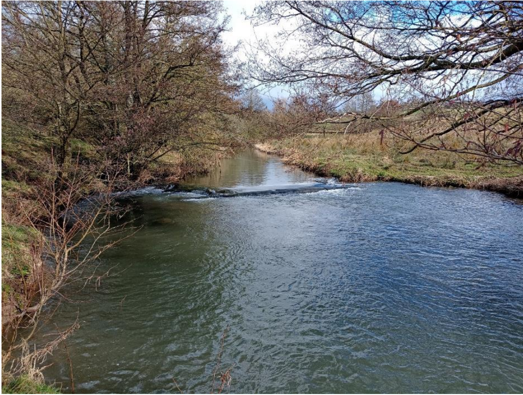
Figure 4 First weir downstream of the ford. Continue to enlarge and deepen the notch close to the true RB (left of shot).
