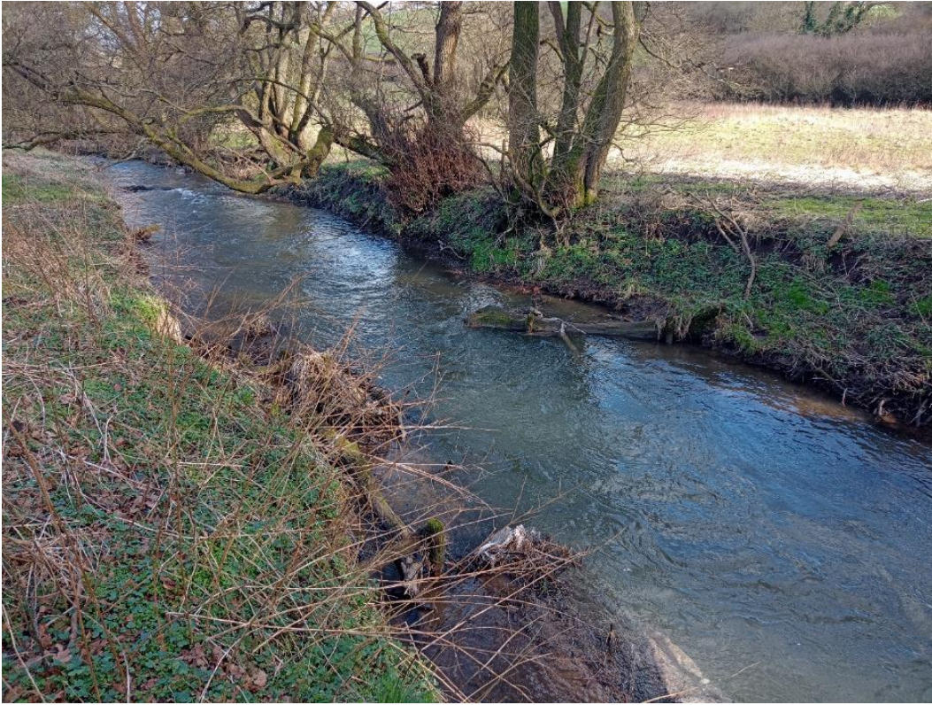
Figure 29 Further upstream from the notched weir, the re-energised flows have allowed previously installed habitat improvements (log deflector, marginal woody cover) to function better. A large amount of accumulated fine sediment has been scoured from this section, increasing depth variability.
