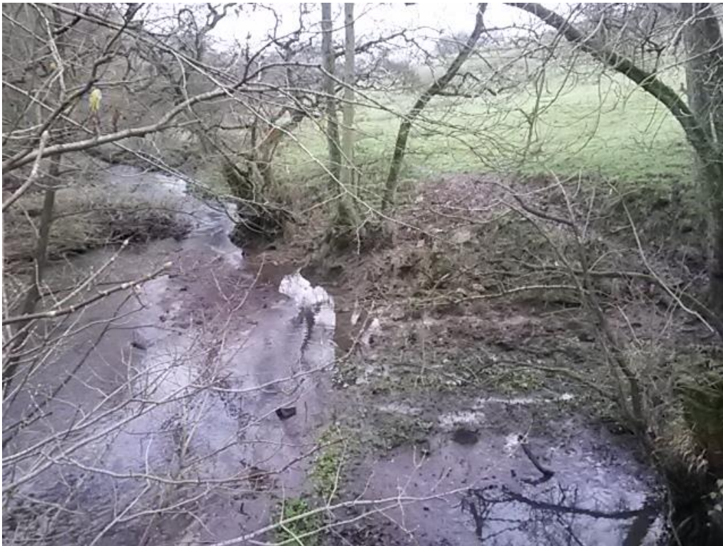
Figure 24 Area downstream of the sluice in 2014 showing typical livestock damage.
