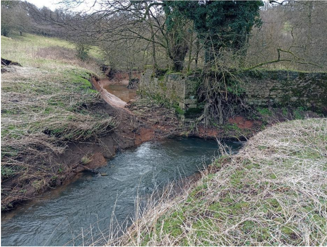
Figure 22 Side channel around the sluice which runs at higher flows.
