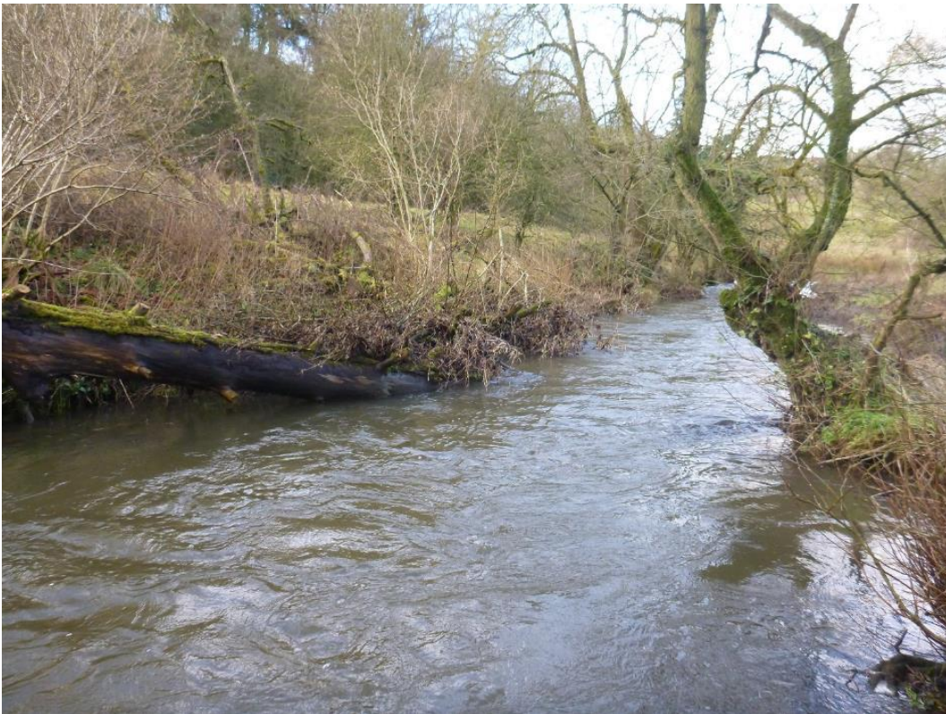
Figure 15 Jan 2016 post-works (completed March 2015). Large trunk winched into the channel and willow & alder trees hinged over to form dense marginal cover.
