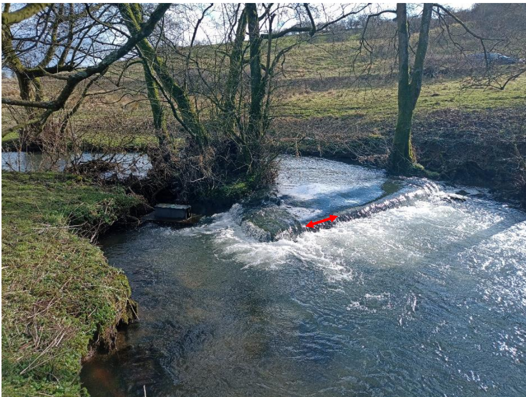
Figure 5 Second weir downstream of the ford. Notch the weir at its lowest point (arrow)
