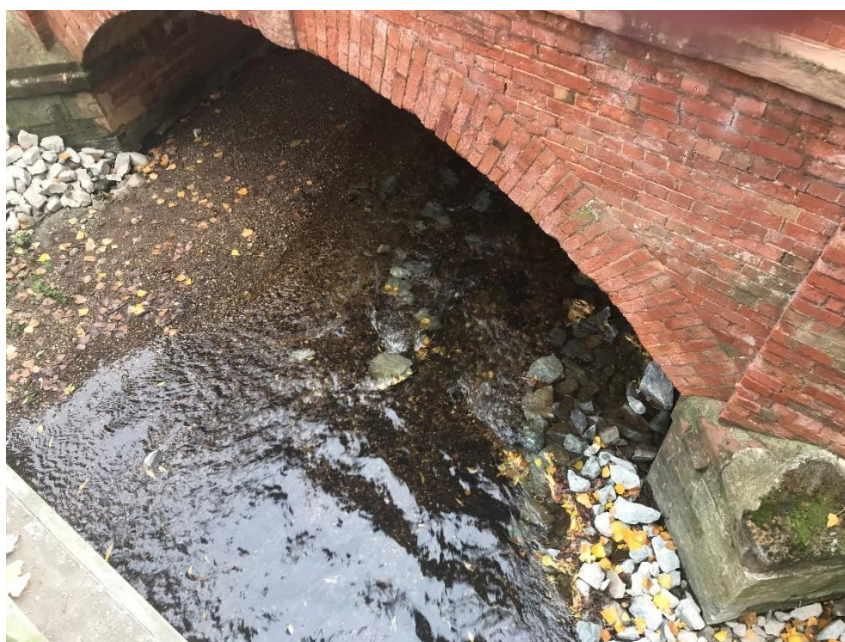
Photo 1 Looking off the footbridge down to the central arch of Gunning’s Bridge. Rip-rap (large, quarried stone) has been placed at the toe of the bridge piers. This isn’t natural but not completely problematic at this location if required, providing some larger structure for a range of aquatic invertebrates to utilise as refuge habitat, along with some of the smaller fish species present.
