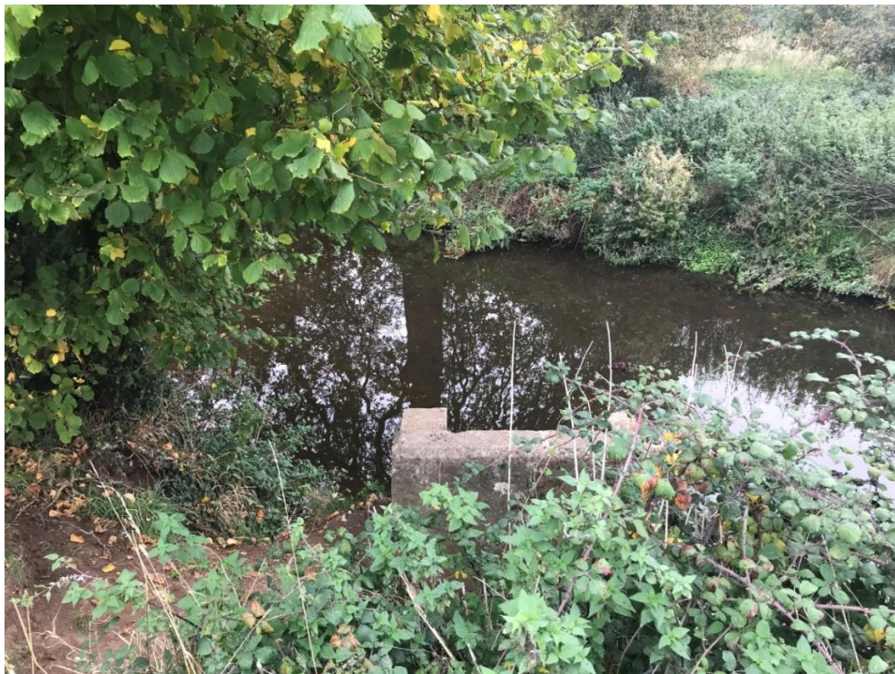
Photo 11 Concrete structure containing the outfall pipe (52.219485 , -1.8716143).
